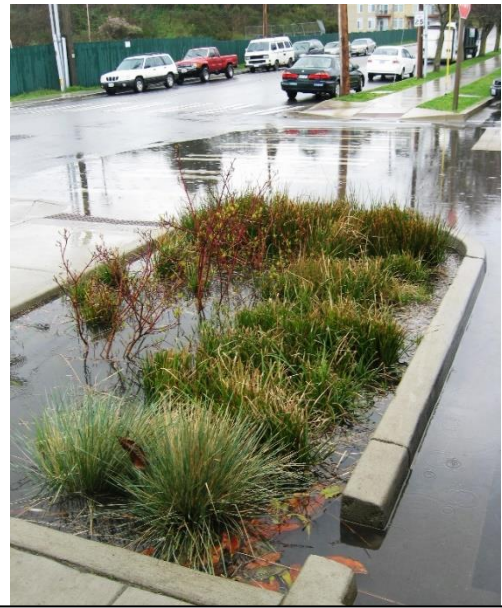
Photo 11: Water can be directed into these cutouts where it will be absorbed by the plants and allowed to percolate.
