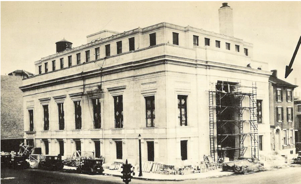
First National Bank and Trust Company in course of construction year 1928. Arrow shows Mr. Reed's home at 604 Cooper St.
