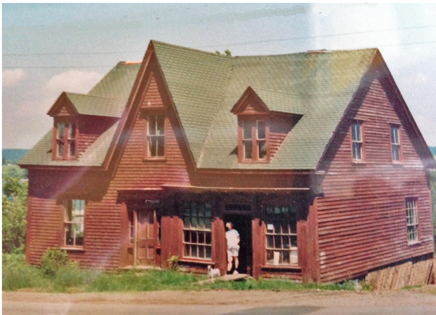
The John Walsh home before the restoration began (courtesy of the author)
