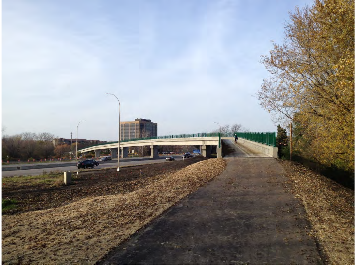
Photo 1: Example Prestressed Concrete Girder Pedestrian Bridge with Decorative Railings
