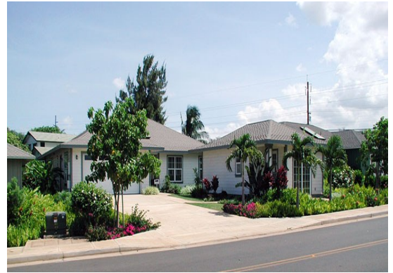
Newly constructed main dwelling and ohana unit in Kihei, Maui
