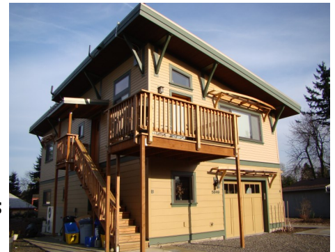
ADU constructed over garage
