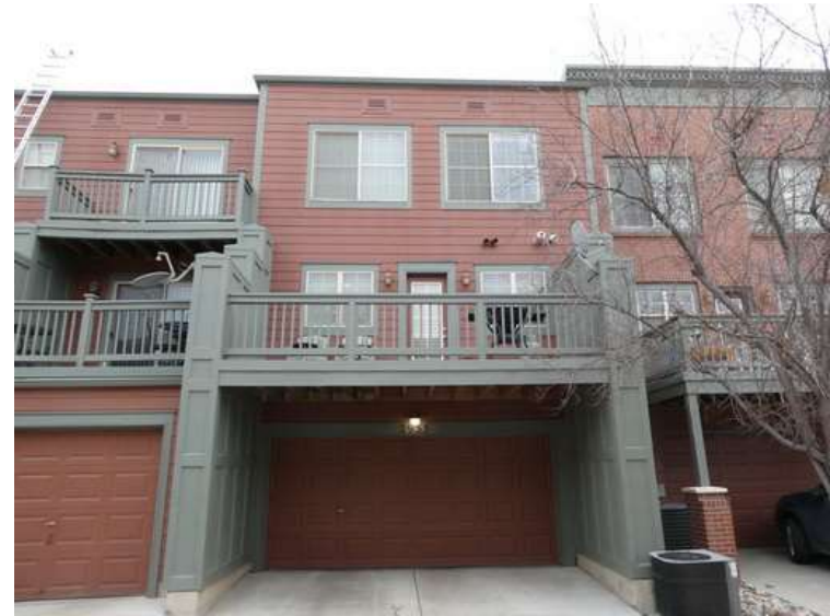
86. Building 03. Unit 2955, west elevation.
