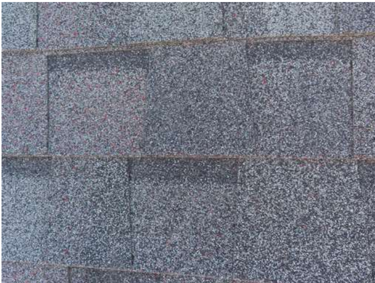
411. Building 18. Typical shingles.
