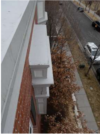
137. Building 05. Painted steel caps.
