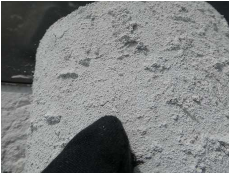
331. Building 14. Tear in the facer sheet adhered to the membrane from hail.
