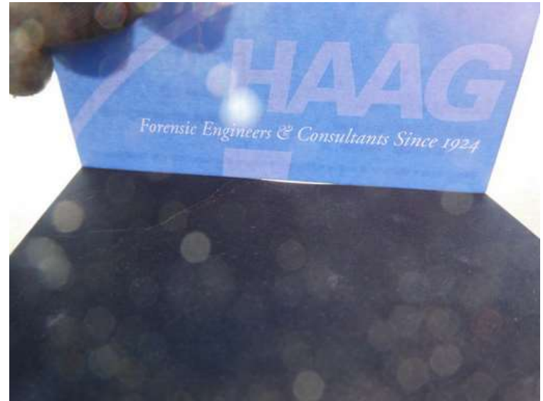
622. Building 25. Straight edge over a dent.
