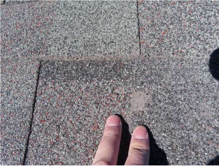
397. Building 17. Mar from installation.
