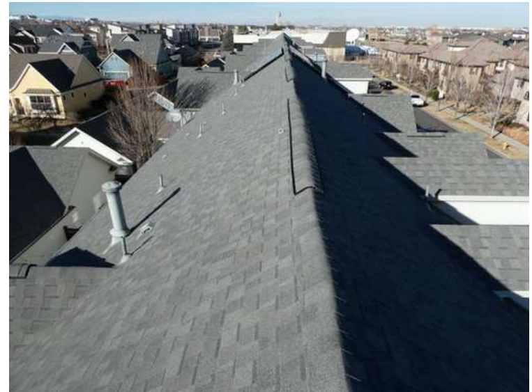
204. Building 08. View looking north.
