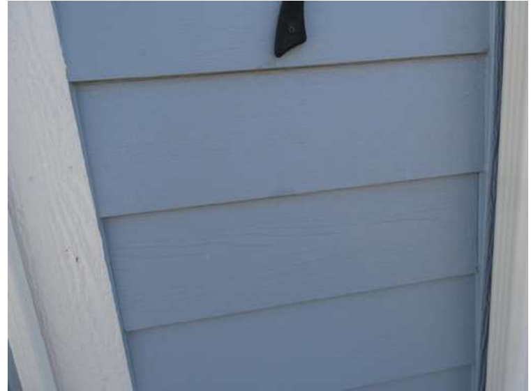
580. Building 24. Paint finishes on siding were not chipped by hail.
