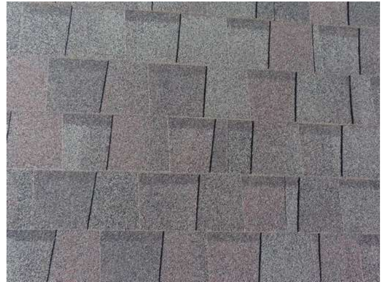
392. Building 17. Typical shingles.
