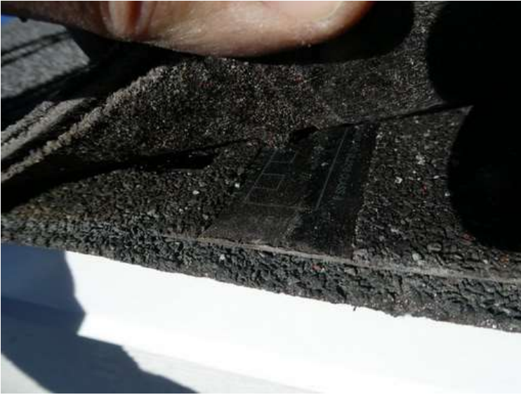
601. Building 24. Cellophane strip indicating Class 4 impact resistant shingle.
