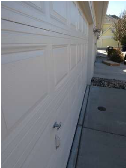
543. Building 23. Garage doors were not dented by hail.
