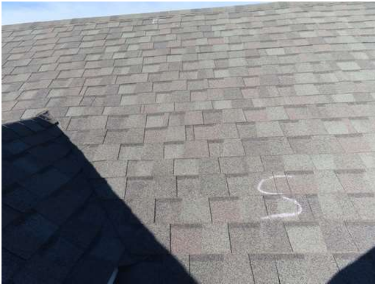
409. Building 18. South test area. No shingles within the test area were bruised by hail.
