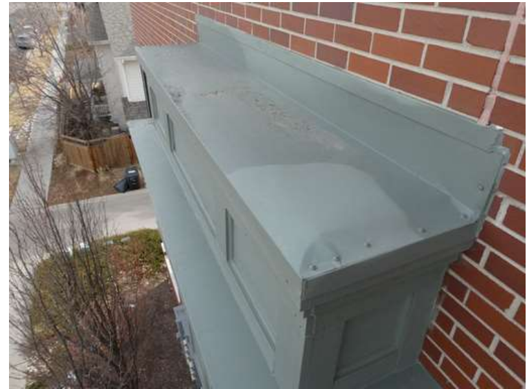
318. Building 14. Painted steel cap.
