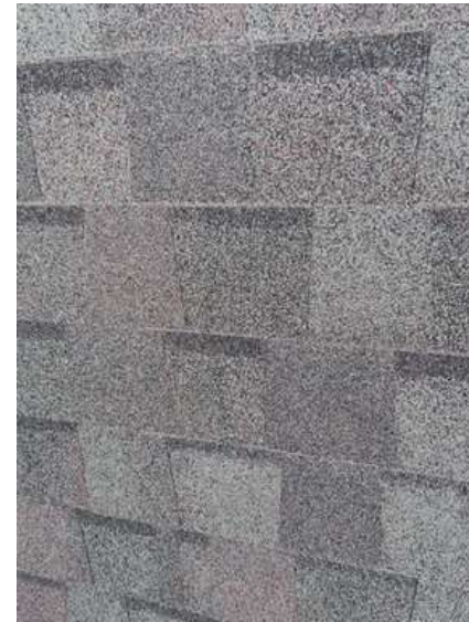
272. Building 11. Typical shingles.
