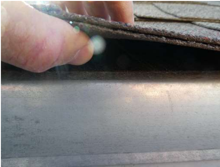
487. Building 21. Ice and water shield.
