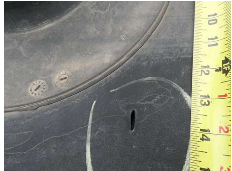
112. Building 04. Mechanical cut.
