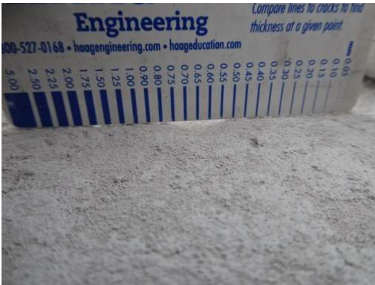
27. Building 01. Straight edge over a dent.
