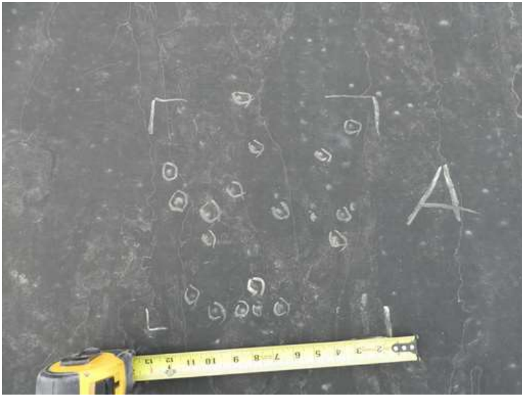
381. Building 16. Test area. Circular chalk marks denote dents in the substrate from hail.
