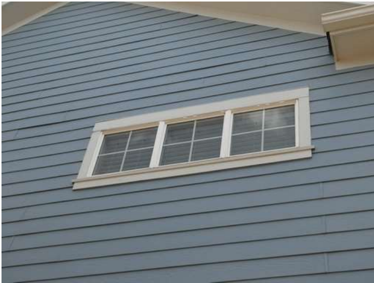
423. Building 19. Another window.
