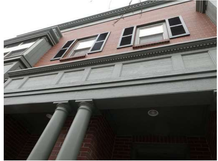
34. Building 02. Panel siding and trim.
