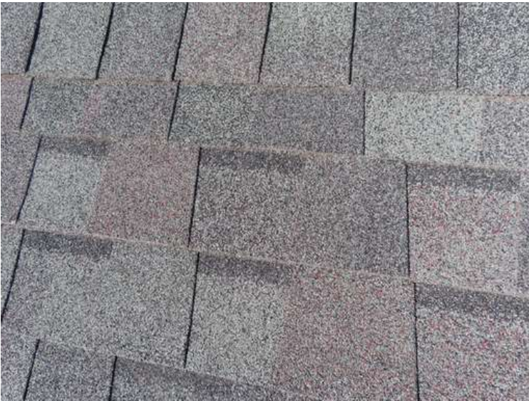
435. Building 19. Typical shingles.
