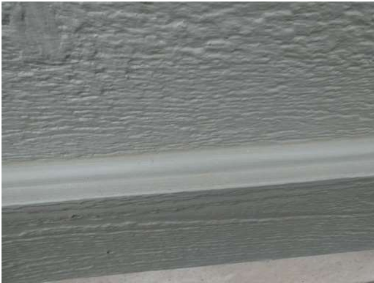
3. Building 01. Paint was not chipped by hail.
