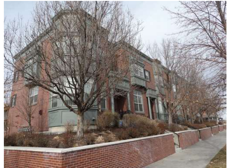
334. Building 15. East elevation.
