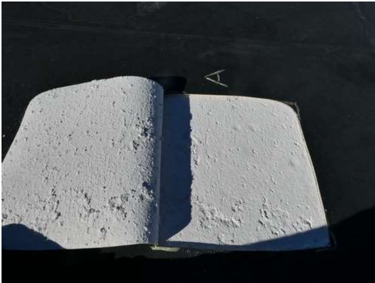
655. Building 26. Sample folded back. The gypsum substrate was dented.
