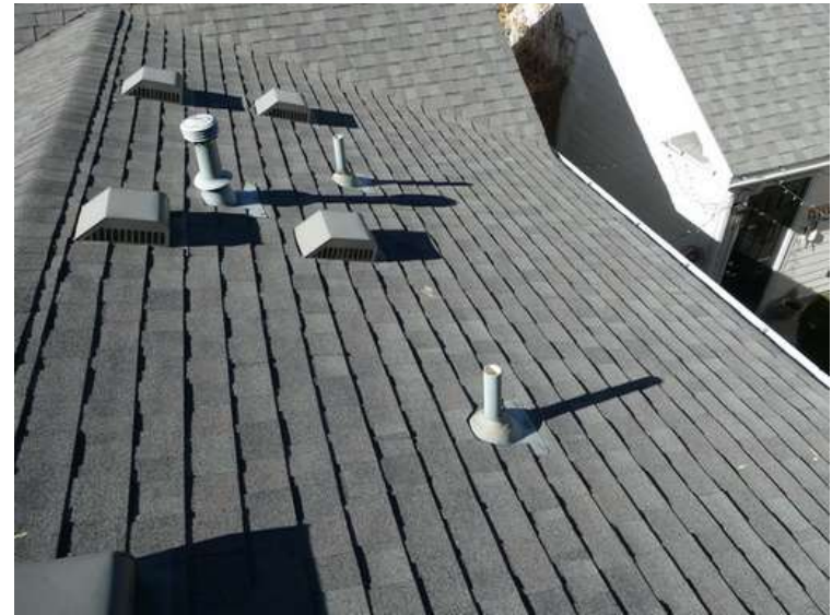
568. Building 23. North test area. No shingles within the test area were bruised by hail.
