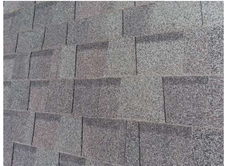
400. Building 17. Typical shingles.
