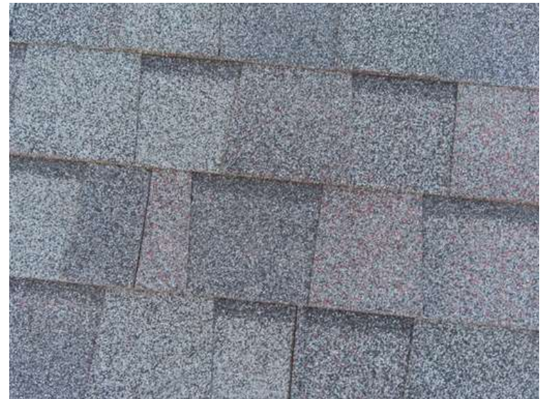
440. Building 19. Typical shingles.
