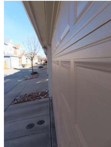
390. Building 17. Garage doors were not dented by hail.
