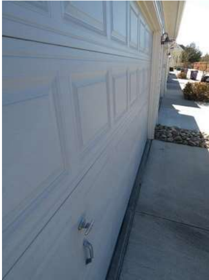
579. Building 24. Garage doors were not dented by hail.
