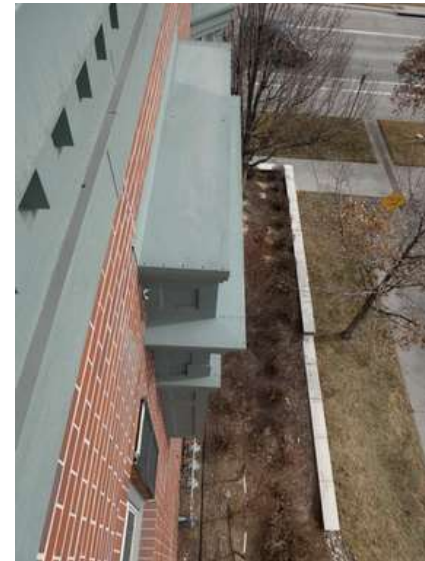
360. Building 15. Painted steel caps.
