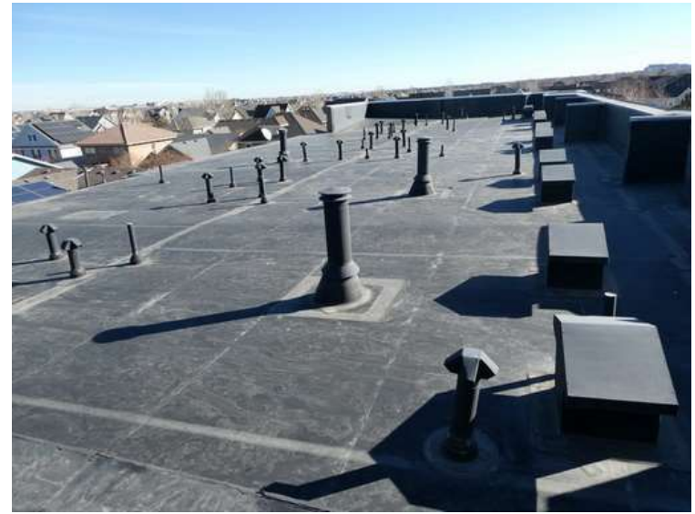
642. Building 26. View looking east.
