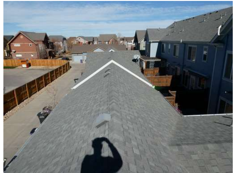
588. Building 24. Garage roofs.
