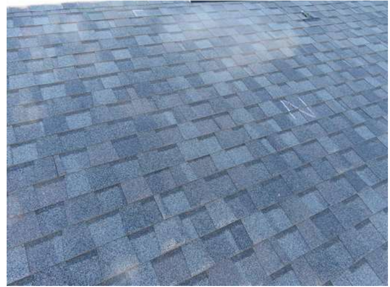
286. Building 12. North test area. No shingles within the test area were bruised by hail.
