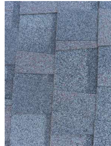
284. Building 12. Typical shingles.
