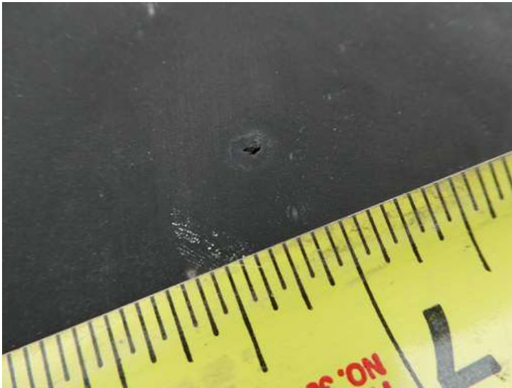
111. Building 04. Mechanical cut.
