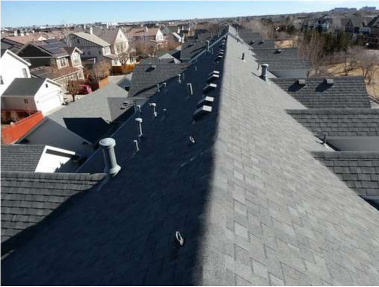
493. Building 21. View looking east.
