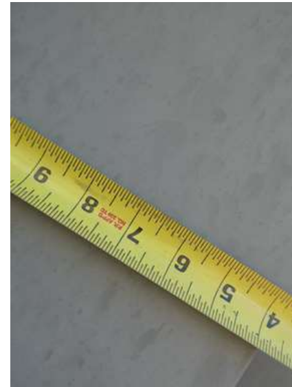
478. Building 21. Spatter marks on an electrical box from hail.
