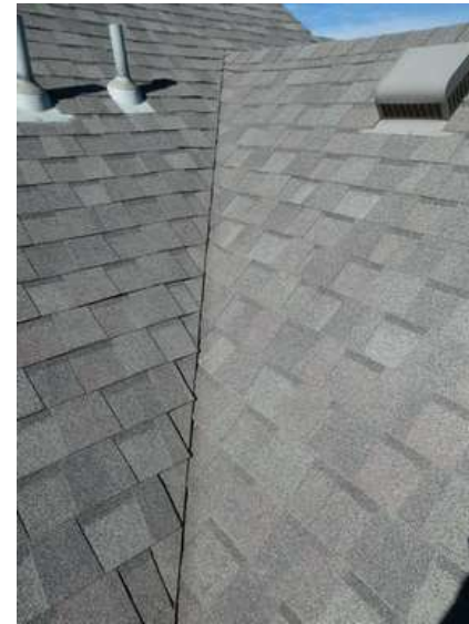
562. Building 23. Shingles draped over valleys were not bruised by hail.
