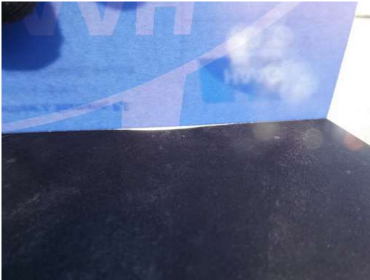
649. Building 26. Straight edge over a dent.
