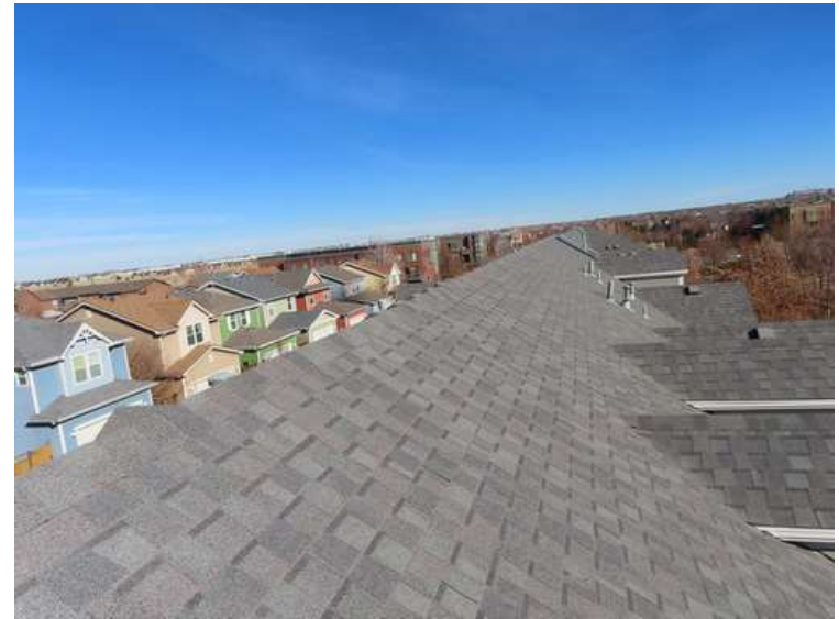
396. Building 17. View looking east.
