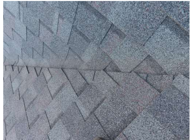
412. Building 18. Shingles draped over valleys were not bruised by hail.
