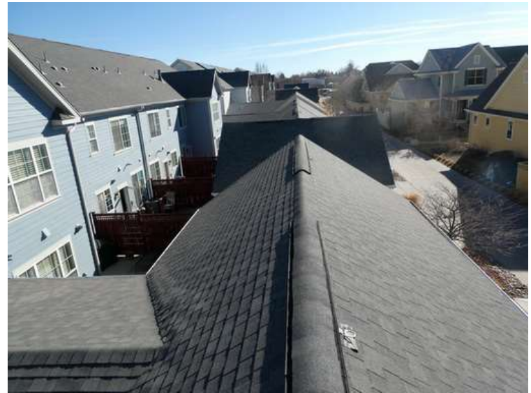
224. Building 09. Garage roofs.
