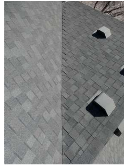
462. Building 20. Shingles draped over valleys were not bruised by hail.
