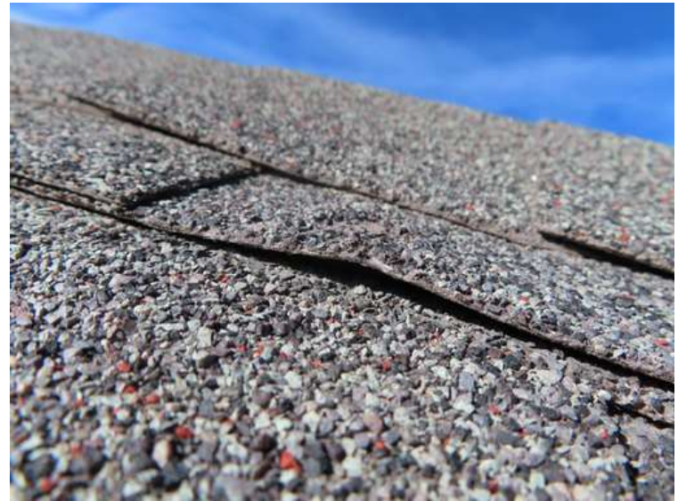
408. Building 18. Another view.
