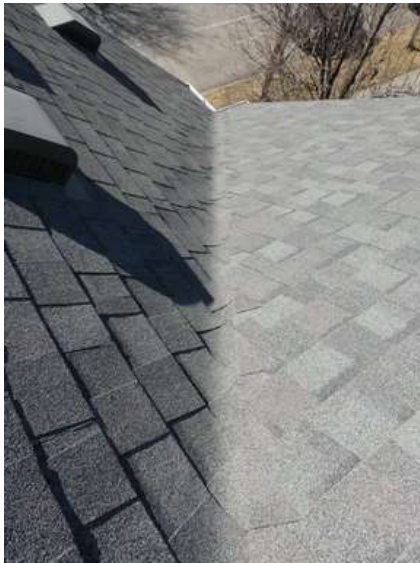
495. Building 21. Shingles draped over valleys were not bruised by hail.
