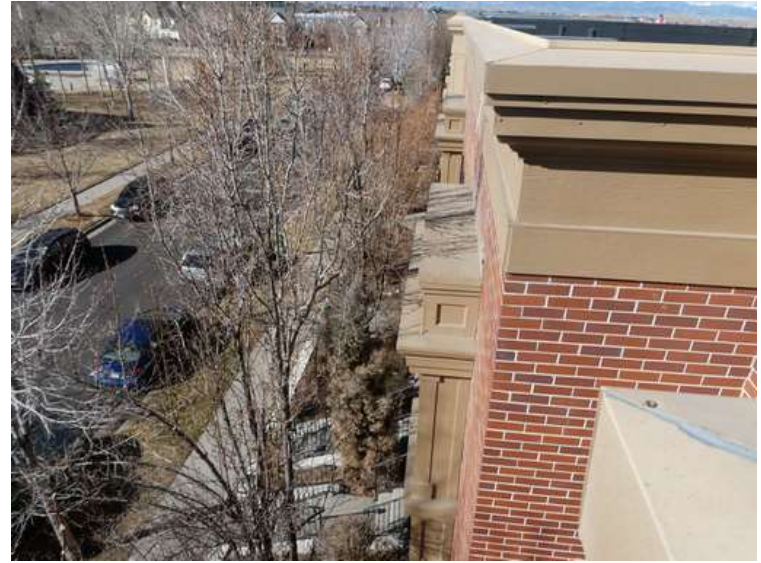
646. Building 26. Painted steel caps on ledges.
