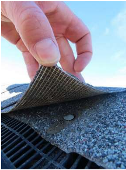
269. Building 11. Extra reinforcements under a ridge shingle.
