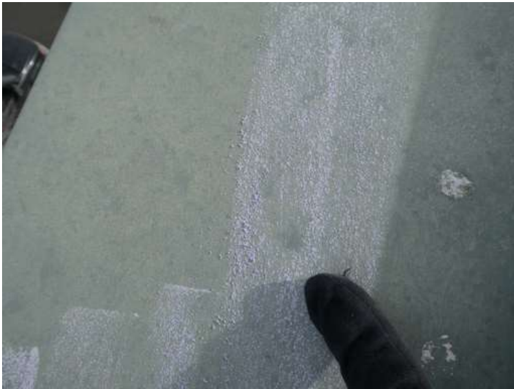
323. Building 14. Dent at a spatter mark.
