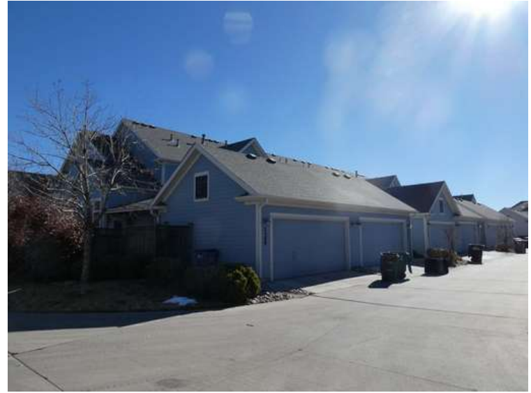
578. Building 24. North and west elevations.
