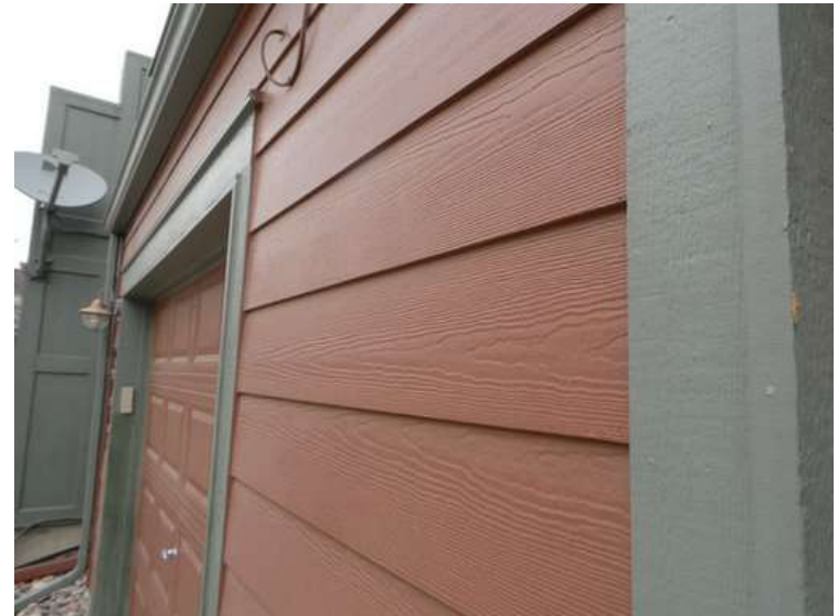
68. Building 03. Paint on siding was not chipped by hail.
