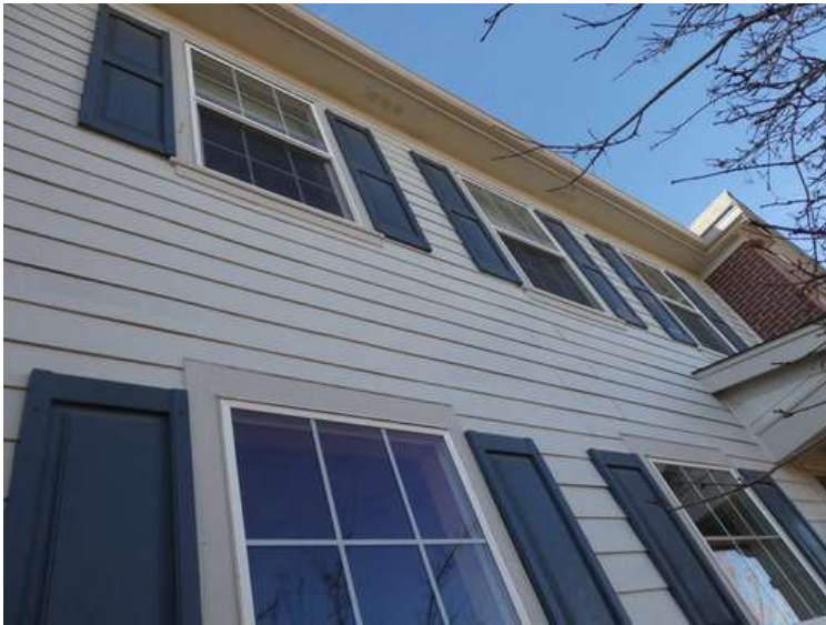
237. Building 10. Paint finishes on fiber cement siding was not chipped by hail.
