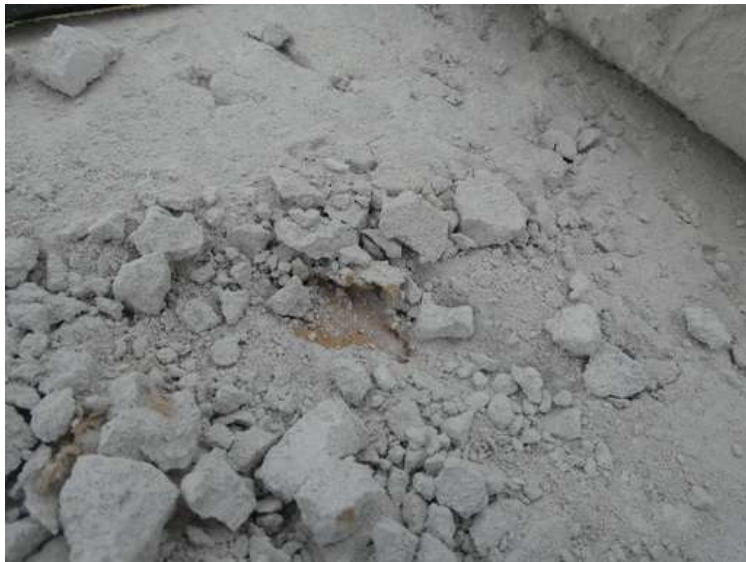
159. Building 06. The roof consisted of a plywood or OSB deck, a layer of gypsum board, and the adhered EPDM membrane.
