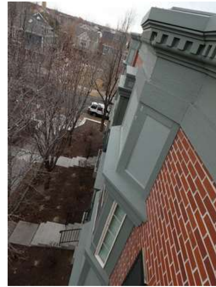
14. Building 01. Ledges of bay windows were capped with painted steel.
