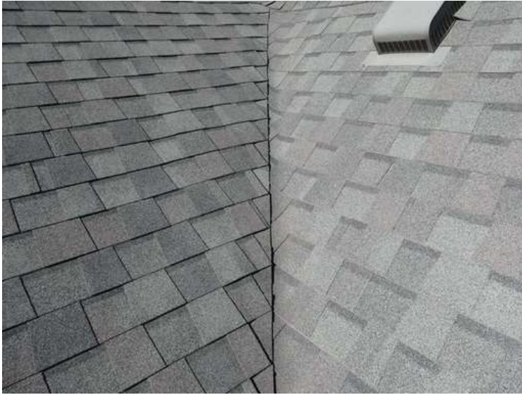
597. Building 24. Shingles draped over valleys were not bruised by hail.
