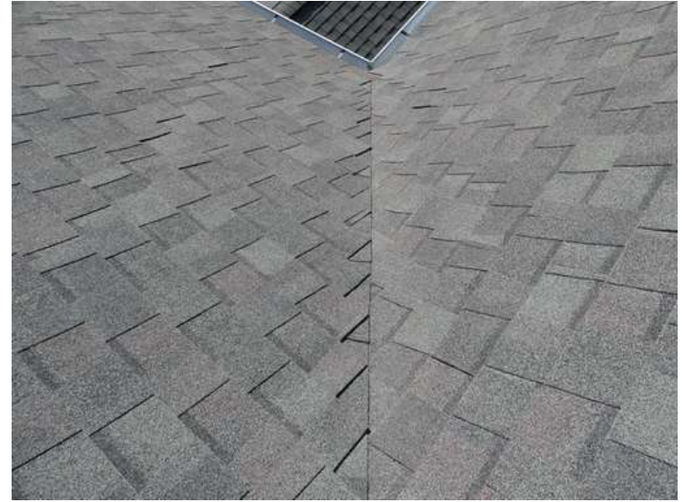
234. Building 09. Shingles draped over valleys were not bruised by hail.
