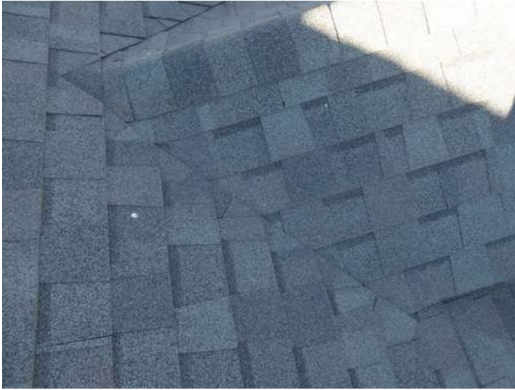
181. Building 07. Shingles draped over valleys were not bruised by hail.
