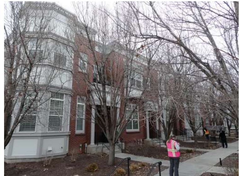
116. Building 05. East elevation.
