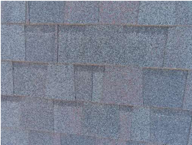
287. Building 12. Typical shingles.
