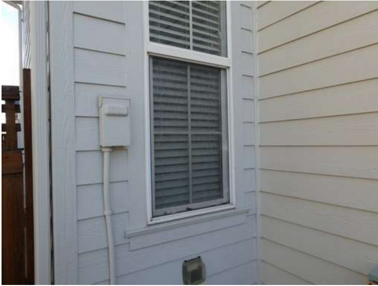
481. Building 21. South window.
