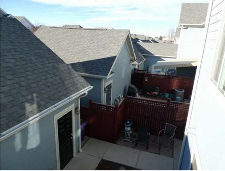
189. Building 07. East elevation of the garages.
