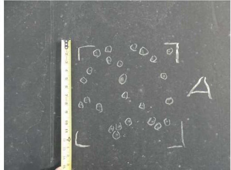
358. Building 15. Test area. Circular chalk marks denote dents in the substrate.
