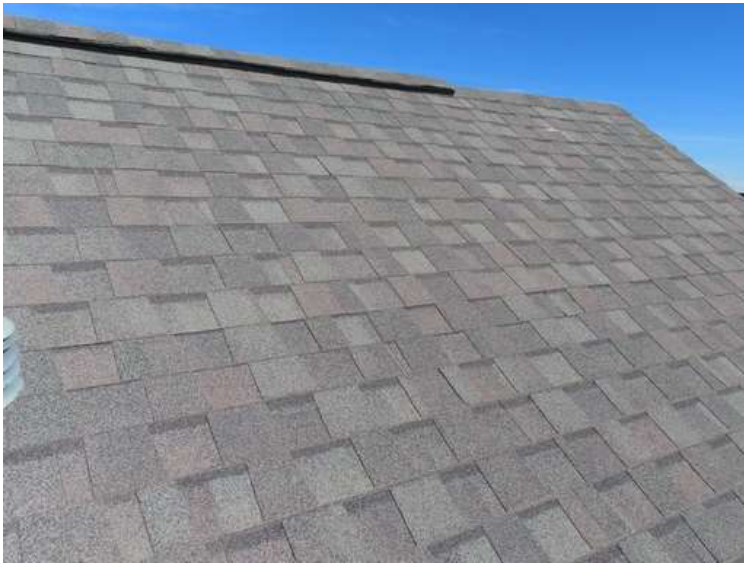
271. Building 11. South test area. No shingles within the test area were bruised by hail.
