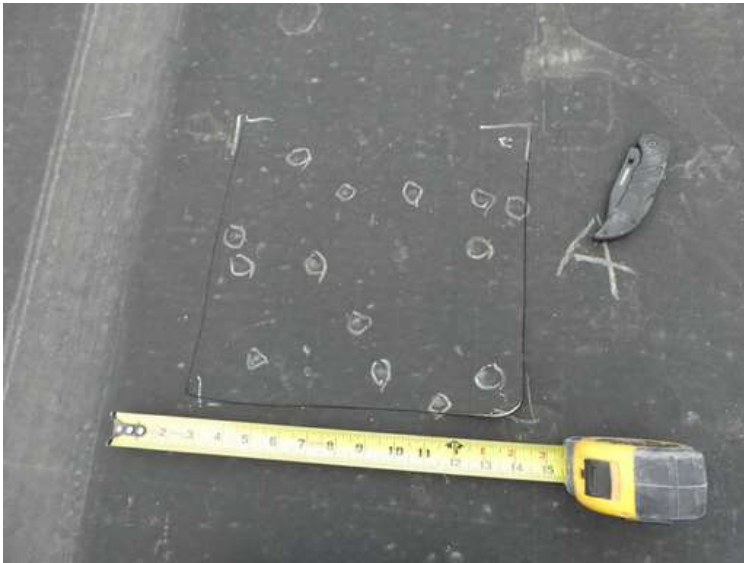
153. Building 06. Sample after cutting.
