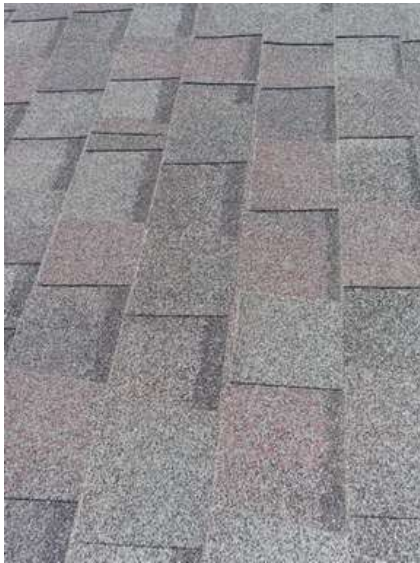
299. Building 13. Typical shingles.
