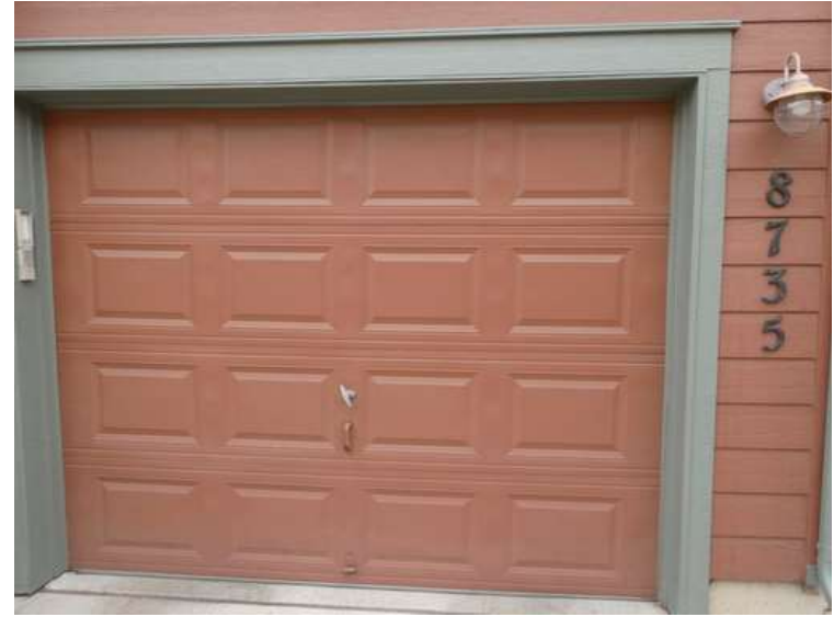
42. Building 02. Garage doors were not dented by hail.
