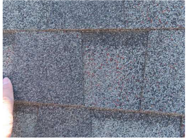
274. Building 11. Typical shingle.
