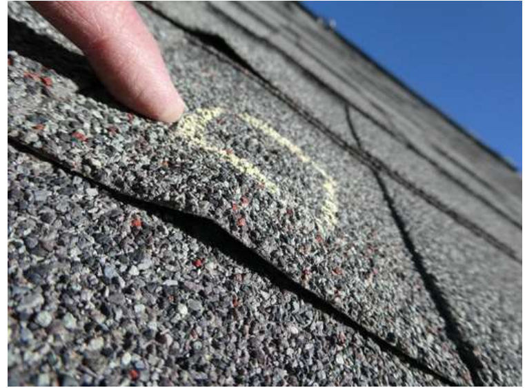
250. Building 10. Another view.
