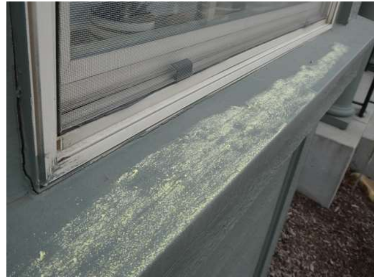
308. Building 14. Dents in metal wall flashing.
