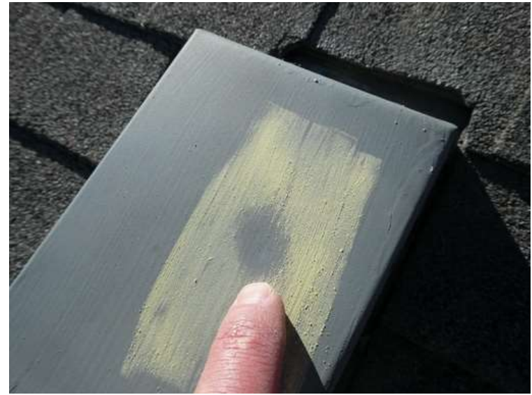
254. Building 10. Dent in an exhaust vent cap from hail.
