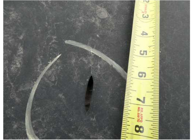
110. Building 04. Mechanical cut.
