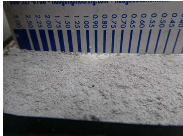
158. Building 06. Straight edge over a dent.
