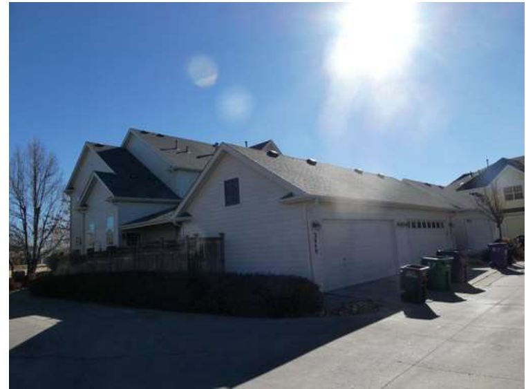
542. Building 23. North and west elevations.
