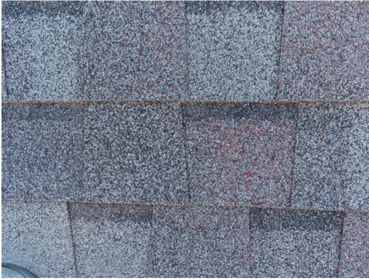
301. Building 13. Typical shingles.
