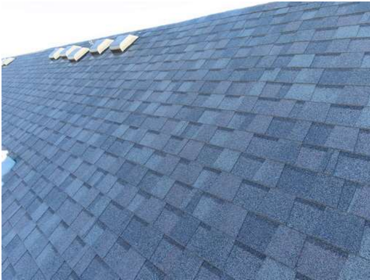
401. Building 17. North test area. No shingles within the test area were bruised by hail.
