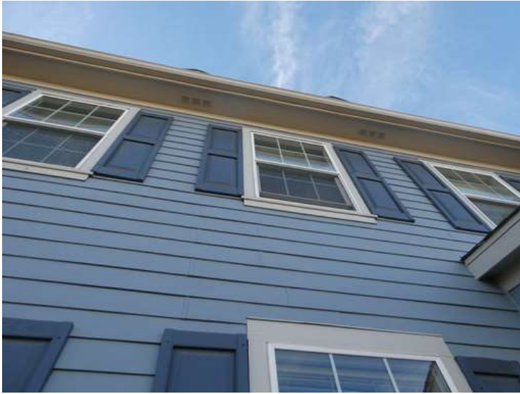
165. Building 07. Paint finishes on fiber cement siding were not chipped by hail.
