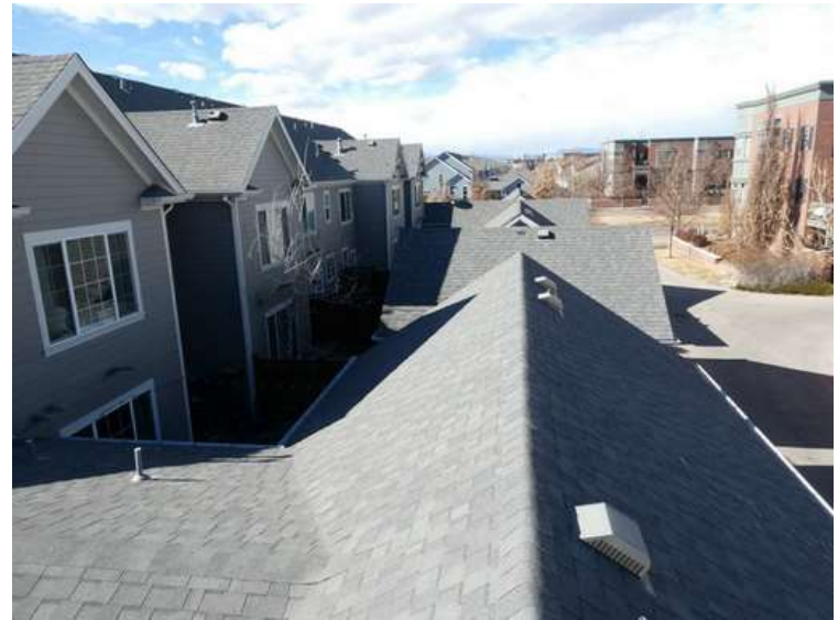
456. Building 20. Garage roofs.
