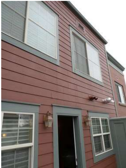
87. Building 03. Perimeter wall.
