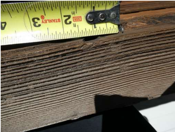
547. Building 23. Dent in a wood fence.
