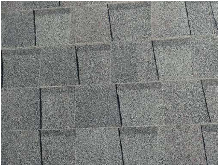
183. Building 07. Shingles were in like-new condition.
