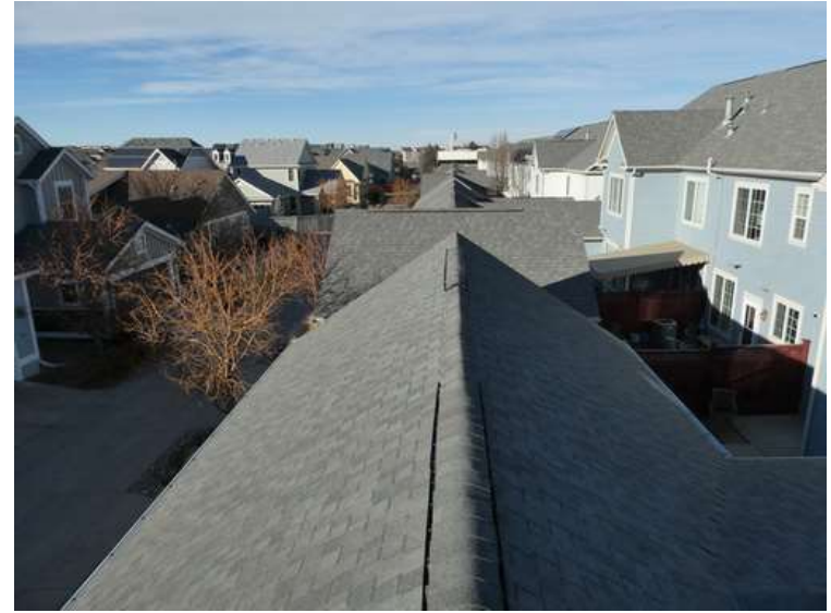
182. Building 07. View looking north at garage roofs.
