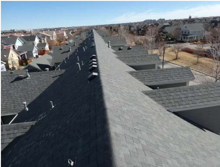
463. Building 20. View looking east.
