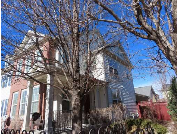
277. Building 12. South and east elevations.
