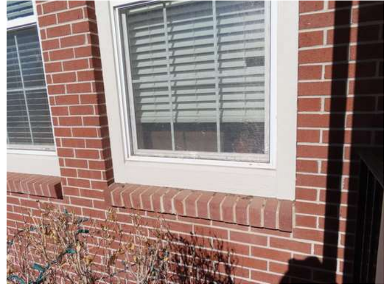
278. Building 12. Tears in a screen.
