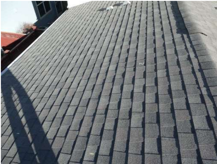
203. Building 08. North test area. No shingles within the test area were bruised by hail.
