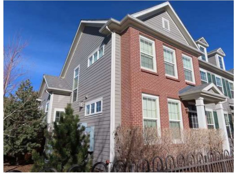
386. Building 17. South and west elevations.
