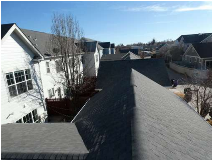
199. Building 08. Garage roofs.
