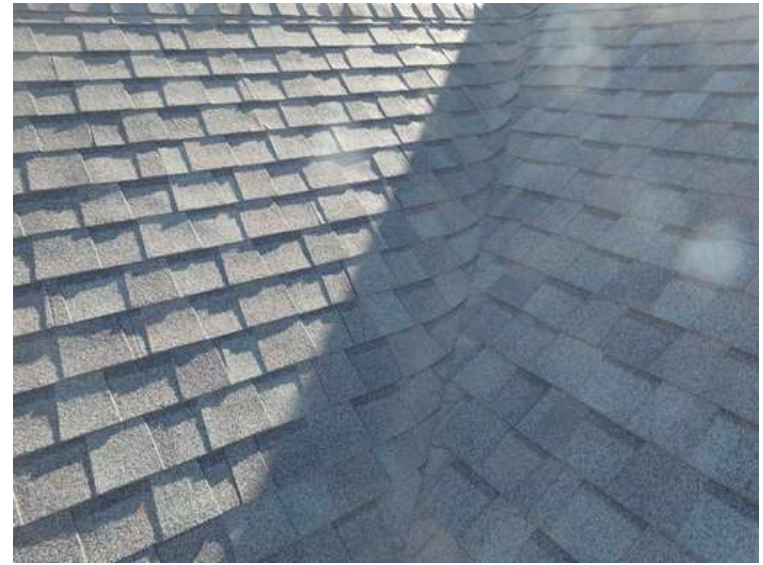
530. Building 22. Shingles draped over valleys were not bruised by hail.
