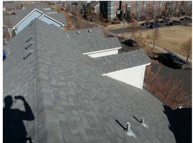
560. Building 23. View looking north.
