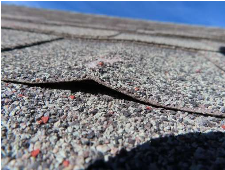
437. Building 19. Another view.
