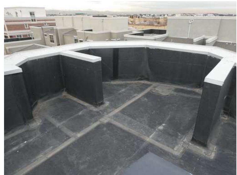
148. Building 06. Parapets with steel caps.
