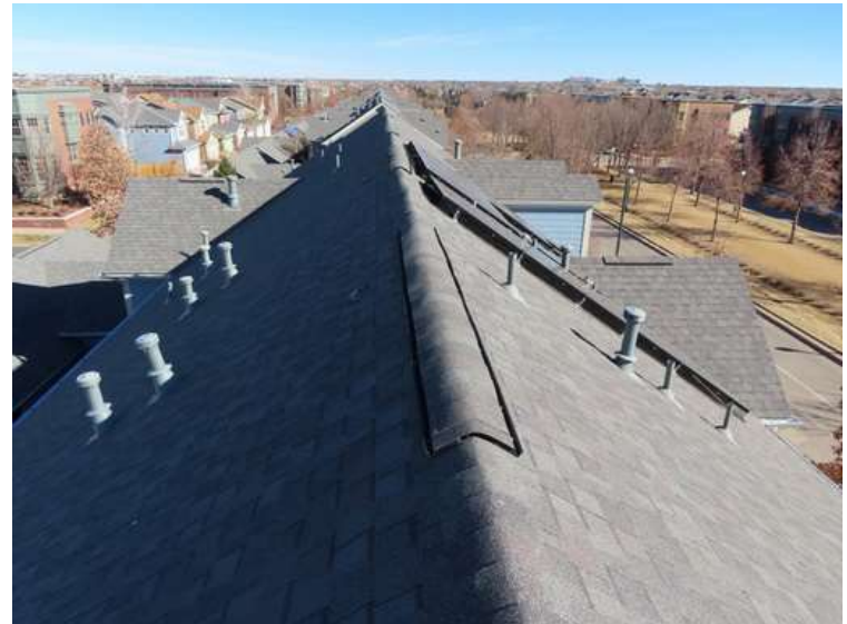
296. Building 13. View looking east.
