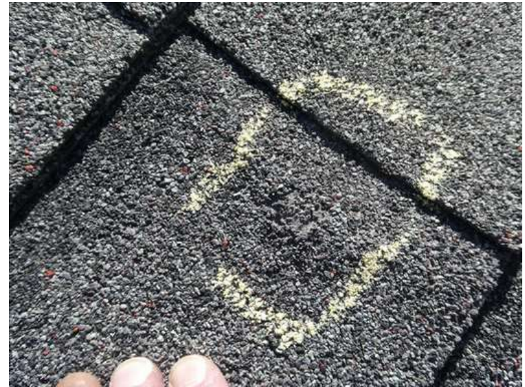
592. Building 24. Closer view.
