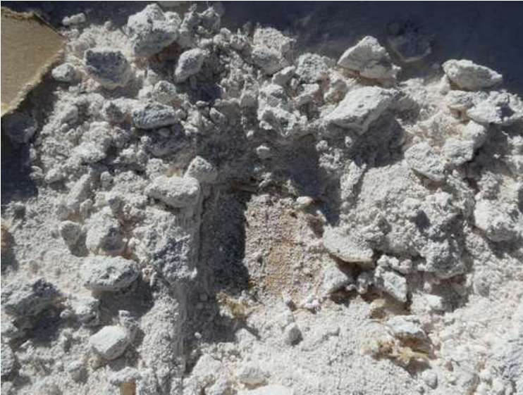
659. Building 26. The roof consisted of a plywood or OSB deck, a layer of gypsum board, and the adhered EPDM membrane.
