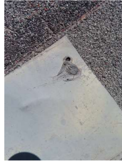
430. Building 19. Re-used flashing.
