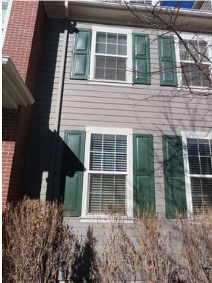
387. Building 17. Paint finishes on fiber cement siding were not chipped by hail.
