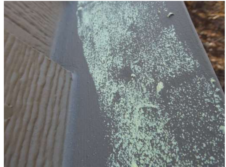
636. Building 26. Dent in a steel ledge.
