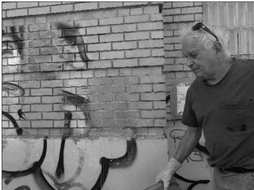
**SANDING MASONRY** surfaces causes damage. Riley Doty comparison-tests paint removal methods at the YWCA.
