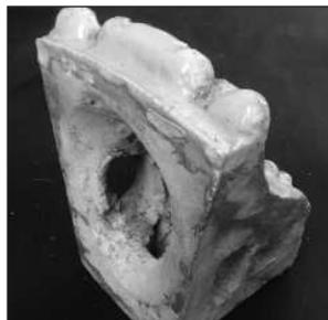
**EIGHT ACANTHUS** leaf units on the Howden Building are just below the center line on the facing of the circular balcony (see page 2). At left, a single piece of a leaf unit, left over from construction in 1925. At right, the hollow cavity is visible at the leaf unit's back. Holes in the side walls were designed to accommodate the metal rod for attachment to the building.
