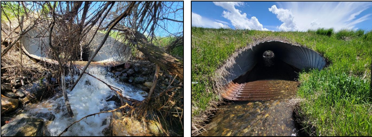
Figure 33 Dry creek culvert outlet (left) and inlet (right).
