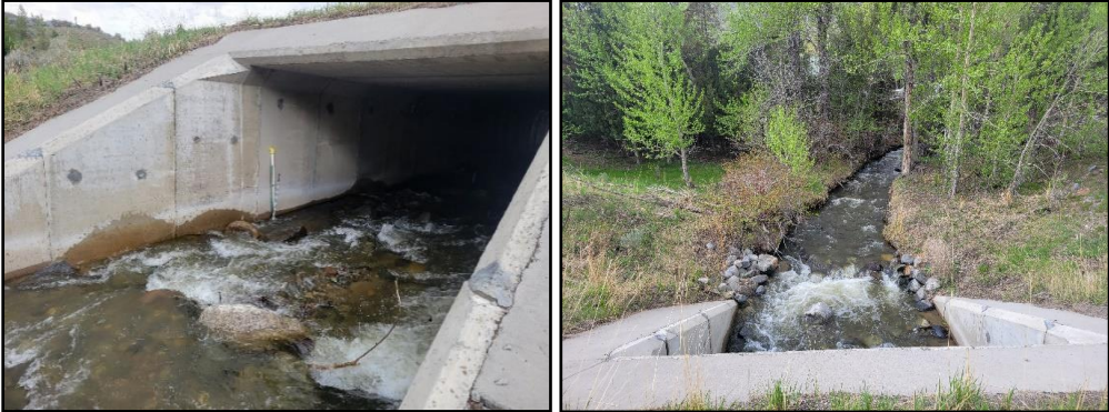
Figure 27 Cedar Creek culvert inlet (left) and stream upstream of culvert (right).
