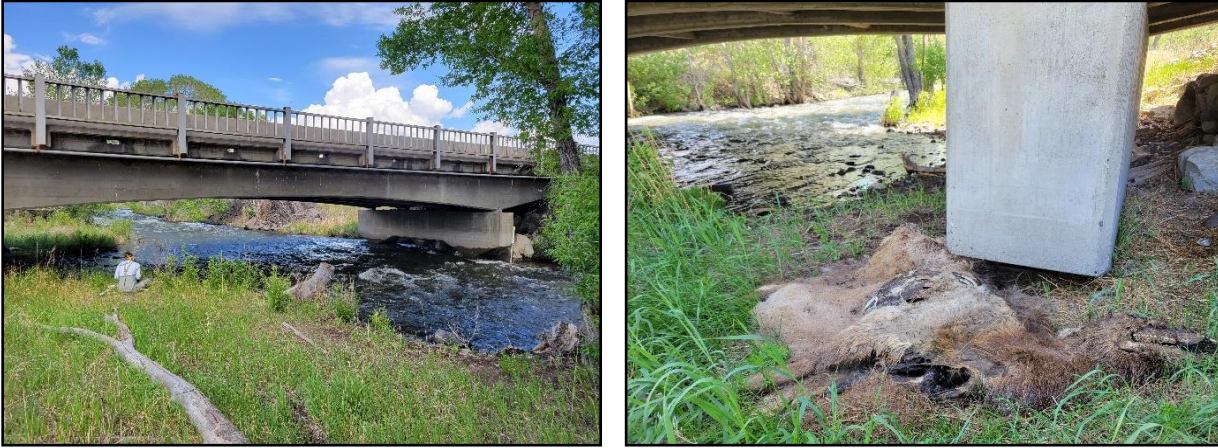
Figure 32 Big Creek Bridge downstream looking upstream (left) and an elk carcass found under the bridge (right).
