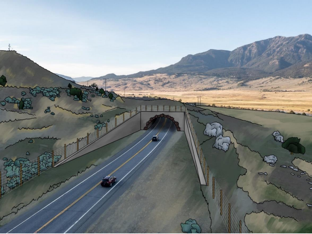
Figure 41. Existing roadway and conceptual rendering of an overpass in the Gardiner Airport Priority Site
