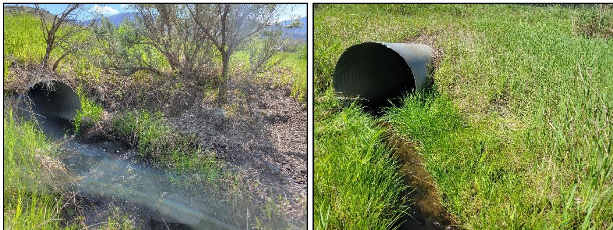
Figure 29 Joe Brown Creek US 89 culvert inlet (left) and outlet (right).
