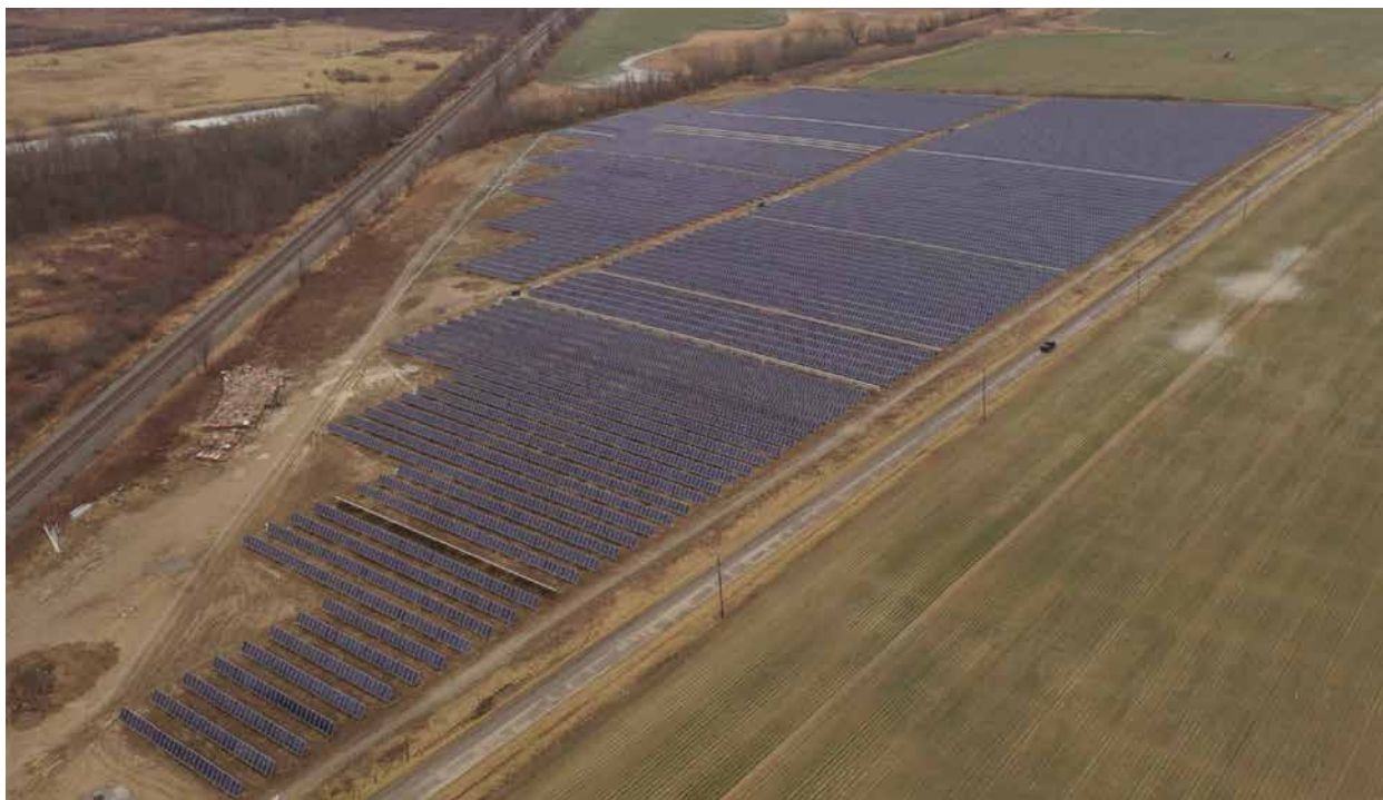
The Village of Grafton receives 10% of its energy from solar power. The 30-year power purchase agreement for this 4-megawatt solar array allows the village to receive energy from the panels at a fixed rate.
