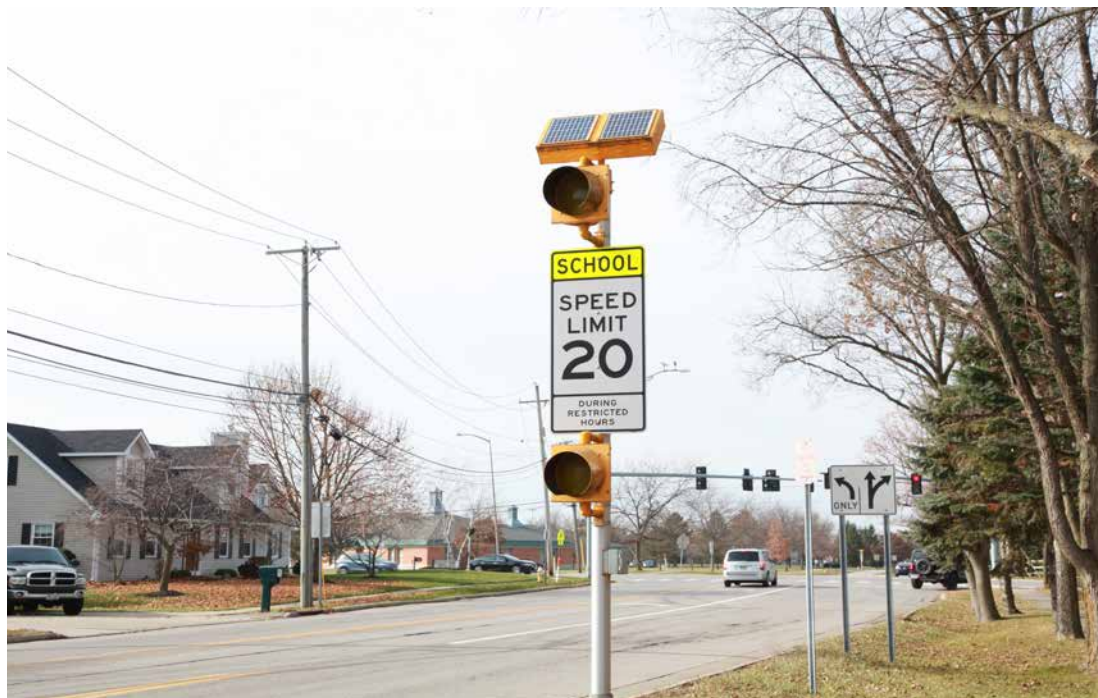
Perrysburg's solar-powered signs and signals are efficient, reliable, and low maintenance. There are cost savings in construction as there is no tear up or stringing to install these signals.
