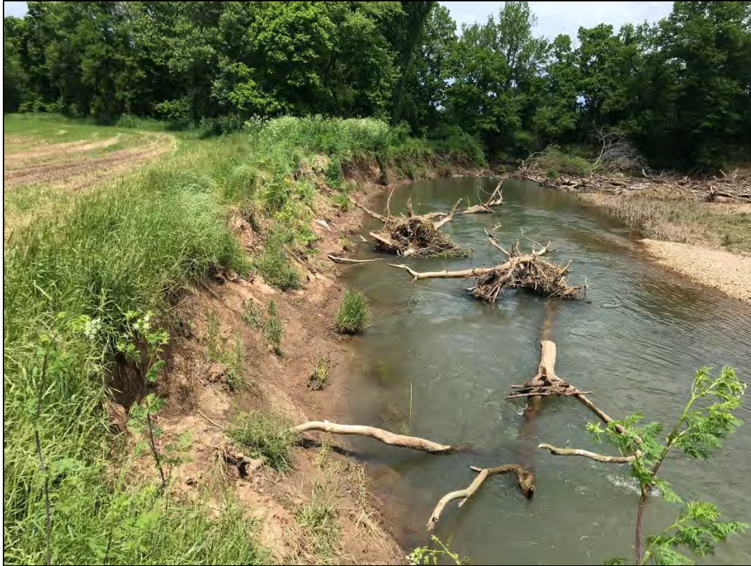
Clear Creek, FID 40 (2019), Downstream View.
