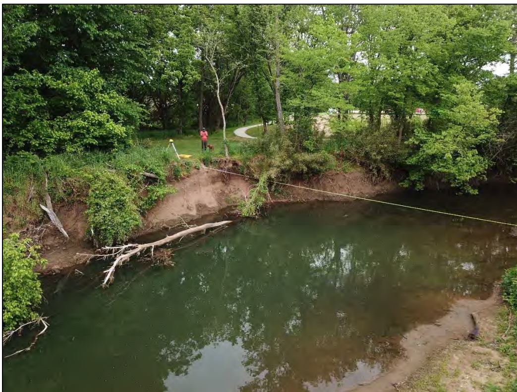
Muddy Fork 1, FID 172 (5/06/2020) Note nearly vertical bank comprised primarily of clay.
