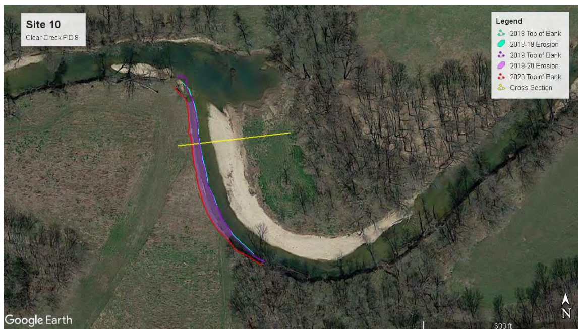
Figure 32. Planform view of Clear Creek FID 8 annual survey site. The area shaded in light blue the location of bank erosion that occurred between the 2018 and 2019 survey dates. The area shaded in purple is bank lost during the time period between 2019 and 2020. Google Earth Imagery Date: 3/4/2020.
