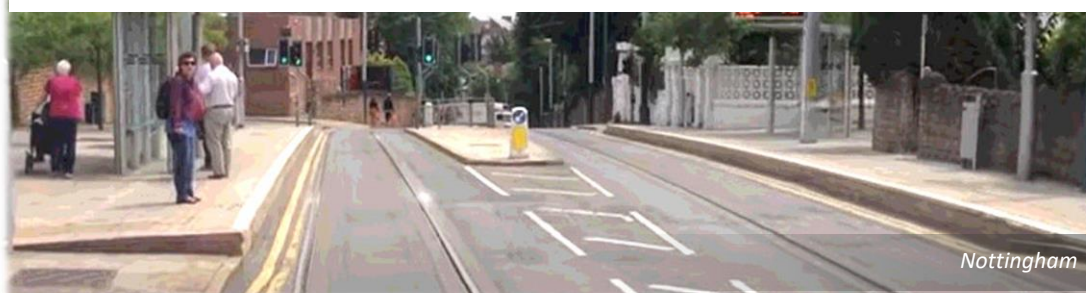
Fig. 23 - Example of a narrow road tram stop. All traffic share, cyclists routed behind tram shelter
