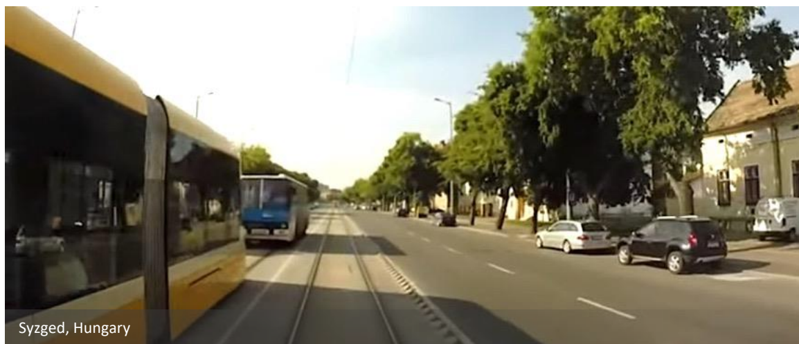
Fig. 10 - Public Transport Pathway (PTP) Tram and Bus track-sharing
