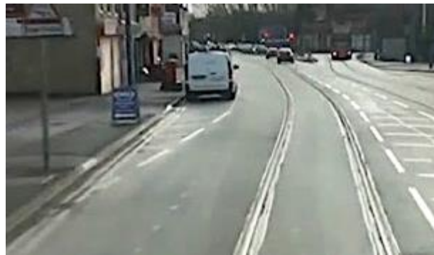
Road space immediately after 'Tram Pinch' re-allocated for delivery vehicles.
