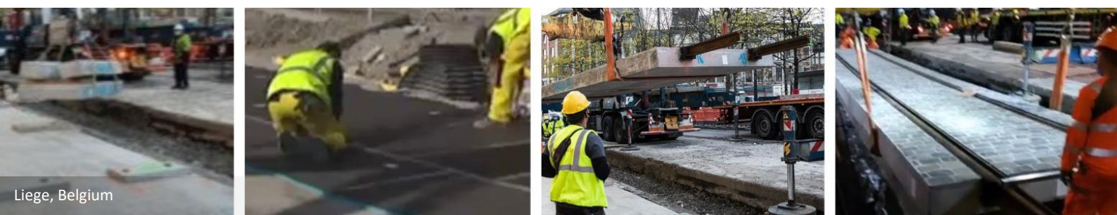
Fig. 2a - Example of a recent track installation process:
