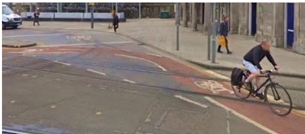
Edinburgh Road Management: "Red Paths" for safe cyclists" to cross tram tracks at a safe angle
