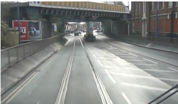
Road Narrows (10.5m) to form a 'Tram Pinch' Midland Metro, Wolverhampton Rd.
