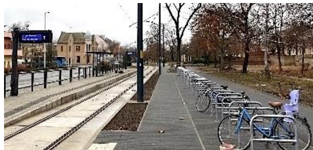
Former three lane road space re-allocated as a bus, tram & bike interchange including Bike + Ride
