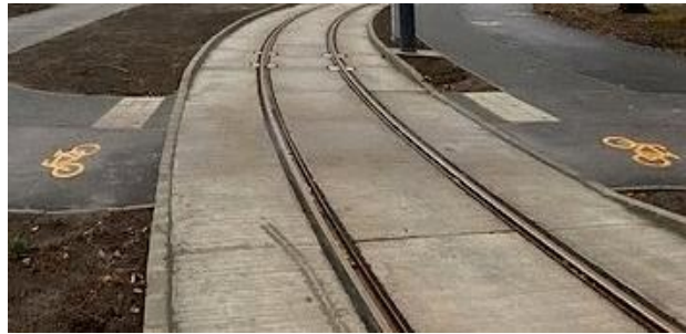
Crossings not less than 45° should be engineered in at time of construction to ensure cycle safety
