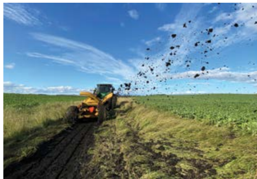
Figure 6. Wolverine ditcher operated by Greenvale Ag Drainage (Photo by R. Wells, Ag Logic)
