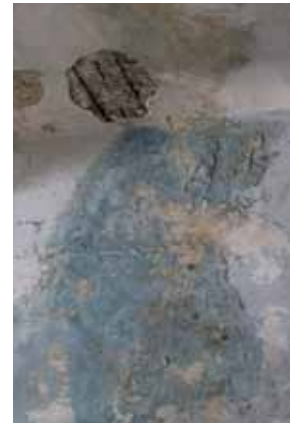
Fig. 9.6 Spalling concrete
