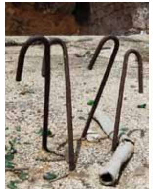
Exposed Rebar
