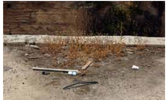
Fig. 9.2 Biological growth at south roofline
