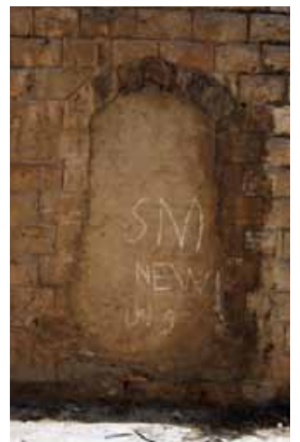
Cementitious Infill Around Doors & Windows
