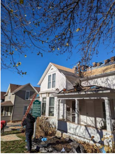
Work begins on Tacy's roof
