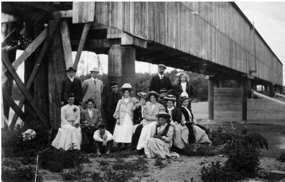
1905 Humboldt Northern covered railroad bridge over Mad River. Photo courtesy of Tom Georgeson.
