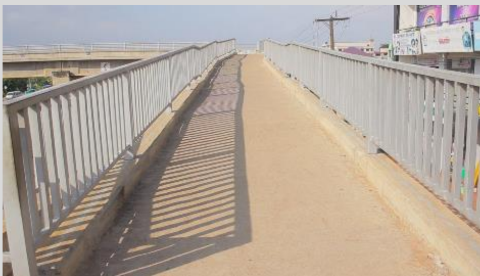
Photo: An accessible footbridge on the Adenta-Madina main road.
