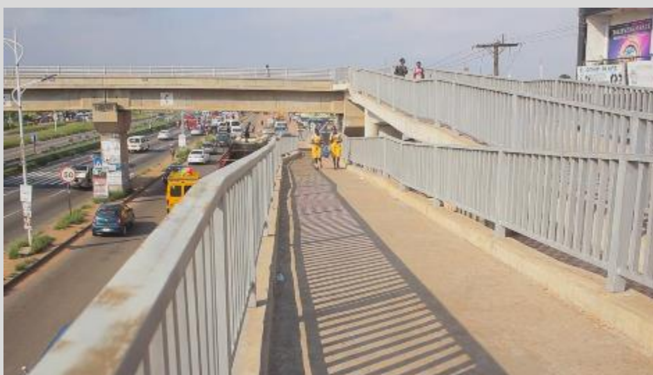
Photo: A gentle slope footbridge on the Adenta-Madina main road.
