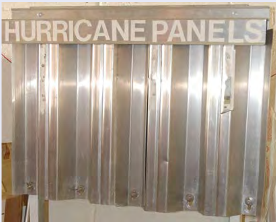
Figure 4-39. Although installation varies, this example shows panels that slip into a track above the window. The bottoms of the panels are secured by bolts that are permanently attached to the window. Photo courtesy of Hurricane Secure.
