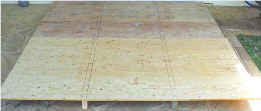
Figure 4-55. During assembly of the shutters in Figure 4-34, the two panels to be joined sit atop the 2 by 4's. The outline of the 2 by 4's and all screw locations are marked on the panel. Panels should be cut, labeled, and marked as to all fastening locations before hurricane season. The panels can be quickly attached with wood screws drilled from the plywood panel into the 2 by 4. The panel is then raised with the end near the window being the pivot point. The panel is then attached to the structural framing of the window as shown in Figure 4-54.
