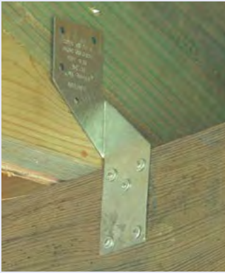
Figure 4-4. This is an example of retrofitting an existing house, originally built without hurricane clips. The popular H3 clip is used here; four nails attach the clip to the roof (truss-rafter) and four more nails attach to the wall or top plate below. For a retrofit, the clips are exposed on the outside of the house. Therefore, both the clip and fasteners should be corrosion resistant and painted to blend with the exterior of the house. With the correct clip and nails, a homeowner could perform the work or hire a licensed contractor. 23
