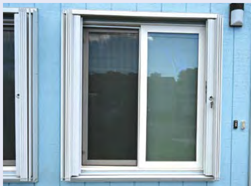
Figure 4-38. For deployment during a storm, the panels unfold accordion-style and extend toward the center of the window along pre-installed tracks. Photo courtesy Hurricane Secure.
