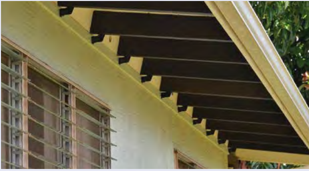
Figure 4-12. With the proper trim, the HPT clips can be installed as shown in Figures 4-7 and 4-8. Every rafter is connected to the wall in an esthetically pleasing manner. Adding trim is not hard to do, but will double the installation time. Two people working on this project can complete the job in 3-4 days.
