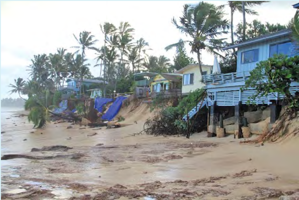
Figure 2-23. Homes on the north shore of O‘ahu in 2013 were threatened by seasonal waves and erosion. Photo courtesy of Dolan Eversole. Many communities are already experiencing impacts from coastal erosion, wave run-up, or flooding, and sea-level rise will exacerbate the problem.
