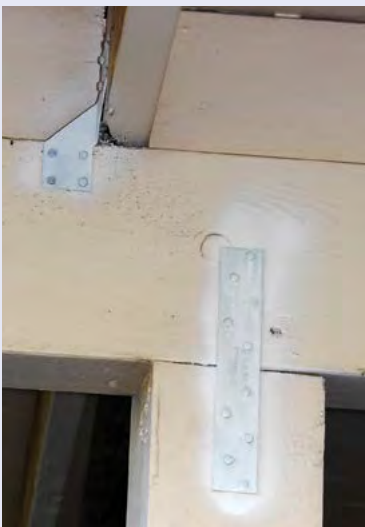
Figure 4-5. In this retrofit example, a hurricane clip attaches the roof structure to a horizontal ridge beam, which is in turn attached to the vertical post with a metal strap. This is an attempt to tie the load from the roof to the foundation, or create the complete load path connection. Note that these clips and straps are in the process of being painted. Photo courtesy of Hurricane Protection Services.
