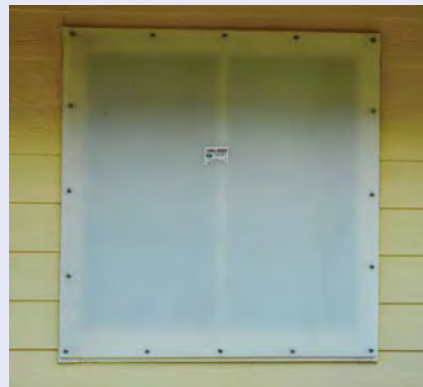
Figure 4-48. In this picture of a plastic honeycomb panel installation, the translucent panel reveals the location of the window to be protected (dark area). The panel overlaps the edges of the window by 4" and the fasteners are in the underlying studs around the window that are part of the structure of the building. A plywood installation would be similar (see Reference Link 47).
