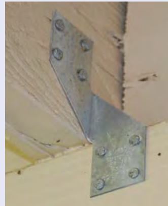
Figure 4-5. In this retrofit example, a hurricane clip attaches the roof structure to a horizontal ridge beam, which is in turn attached to the vertical post with a metal strap. This is an attempt to tie the load from the roof to the foundation, or create the complete load path connection. Note that these clips and straps are in the process of being painted. Photo courtesy of Hurricane Protection Services.
