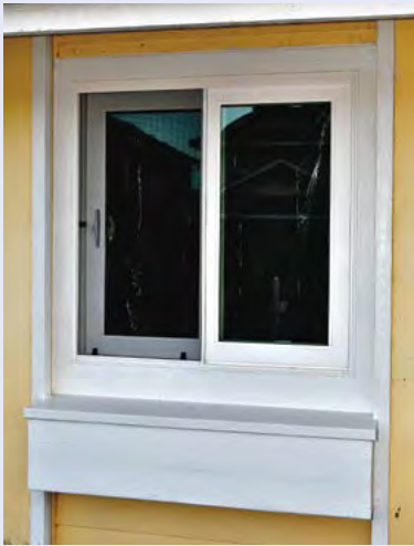
Figure 4-41. This impact-resistant window is installed on a typical double-wall house on O‘ahu. This window has passed the ASTM E 1996 standard, Missile “D” 9.0 lb 2” x 4” at 50 ft/sec or 34 mph. The advantage of this system is that it is always in place to provide year-round protection against hurricane wind-borne debris, or a robber. In addition, there are environmental sustainability and climate adaptation benefits related to reduced sound, protection from damaging UV radiation, reduced heat intake, increased views and privacy (see box). Photo courtesy of Coastal Windows.
