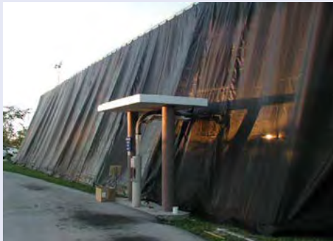
Figure 4-43. Hurricane screen, mesh, or fabric consists of woven polypropylene or a resin coated ballistic nylon. The screen can cover large areas and provide protection to windows with unusual configurations. Light can pass through the fabric so that the area inside is not totally dark. Photo courtesy of the Department of Emergency Management, City and County of Honolulu.
