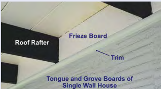
Figure 4-9. In this more difficult installation, the molding needs to be removed and replaced with a trim board so that the 1.5 inch screws don't penetrate through the wall of the single wall house, which is typically \frac{3}{4} to 1\frac{1}{8} inch thick.
