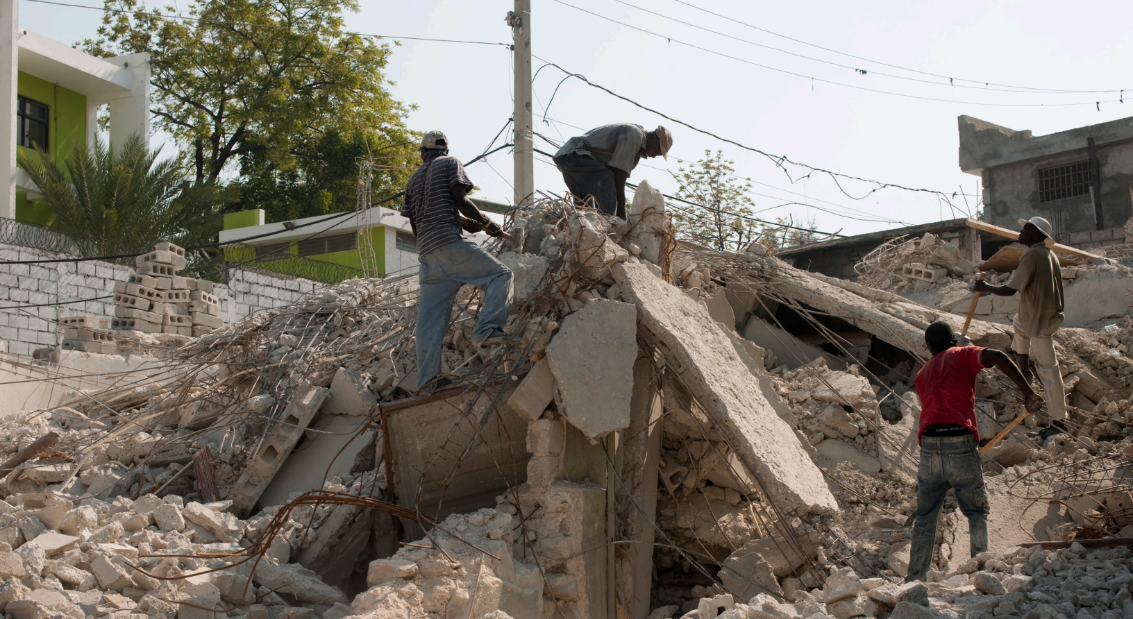
Men look for survivors in a collapsed building after the 2010 earthquake.
