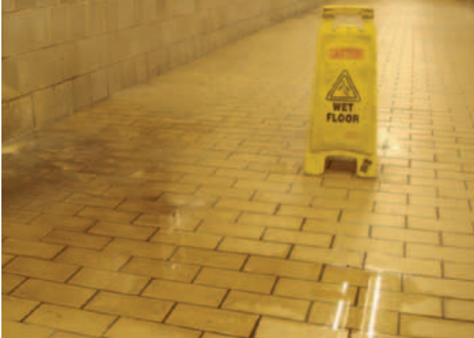
Wet slippery floor
