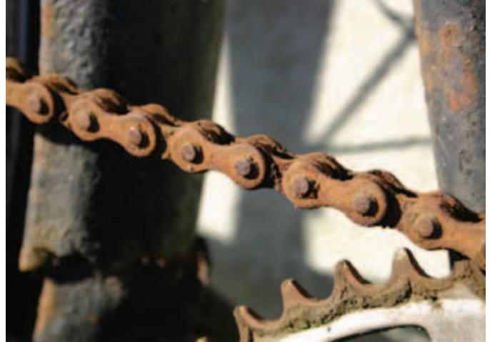
Old, Broken or Unguarded Equipment
