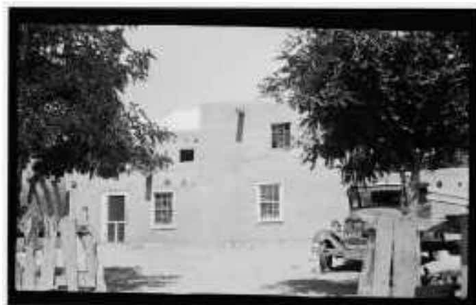
Caretakers House- Ranchos de Taos Plaza, August 1936 Vigas dated to 1774-75. This house may have been built into the defensive wall of the Plaza. Photo: Frederick D. Nichols
