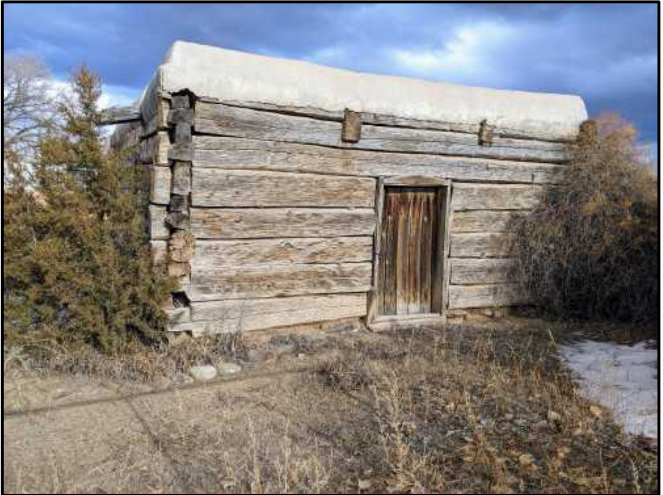
Hewn log fuerte, built by Alfredo Santistevan in 1888, La Cordillera Photo: Hank Saxe
