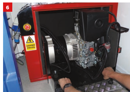
6) Now fully removed, Engine/ Alternator can be worked on
