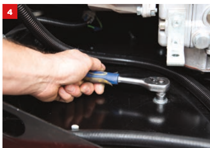
4) Remove x4 bolts (x2 bolts on Redbox Infinity) holding the genset carrier to the Enclosure
