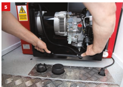
5) Pull Engine/Alternator carrier out using the handles provided
