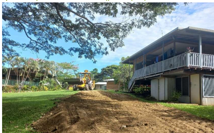
Work has commenced on a home for the Slaa family at RCBC in Port Moresby
