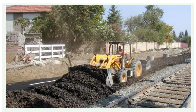
Tire-derived aggregate from recycled scrap tires can help reduce vibration and noise from trains.
