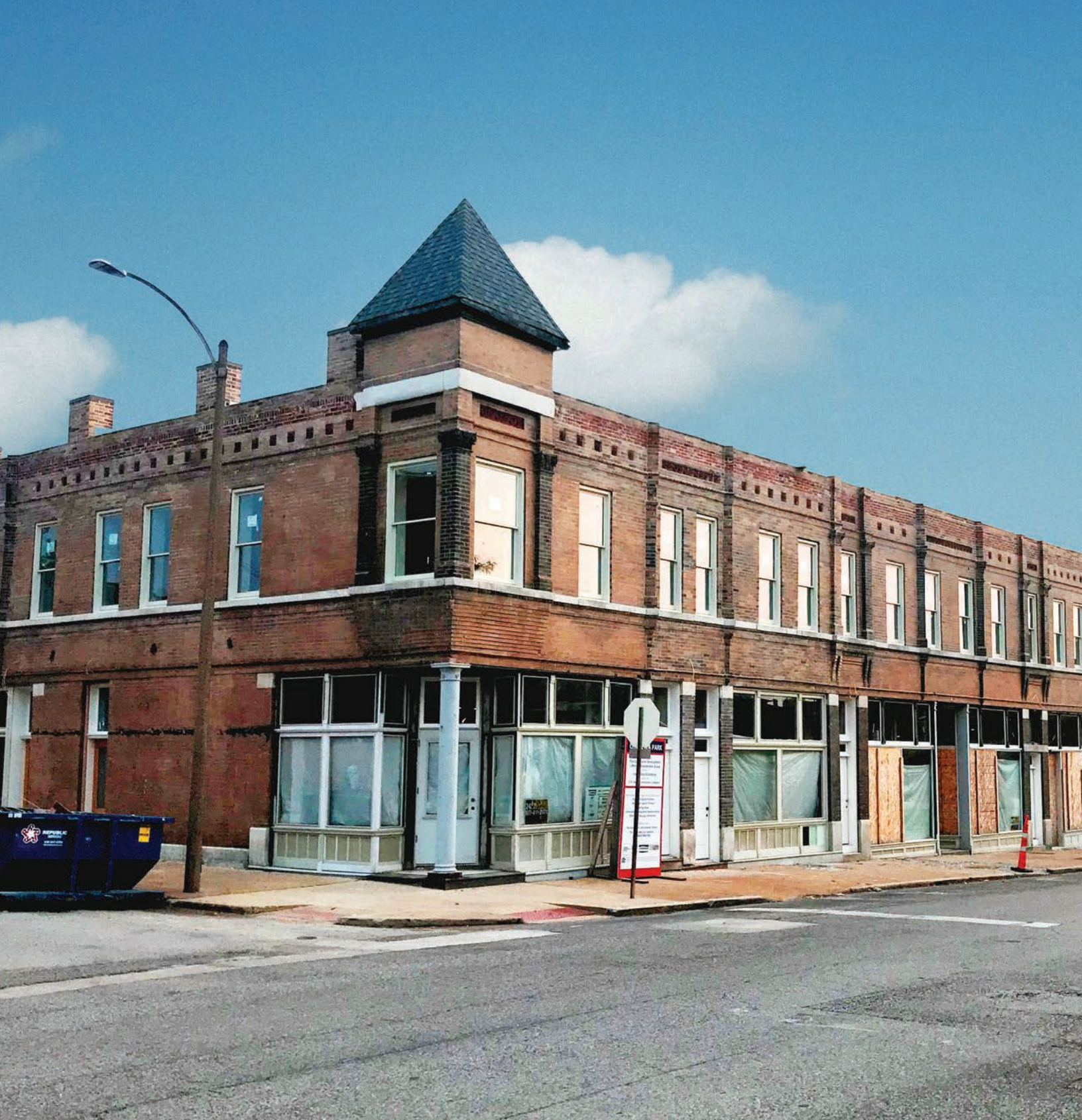
Photo of new rehab for affordable housing on Chippewa.
