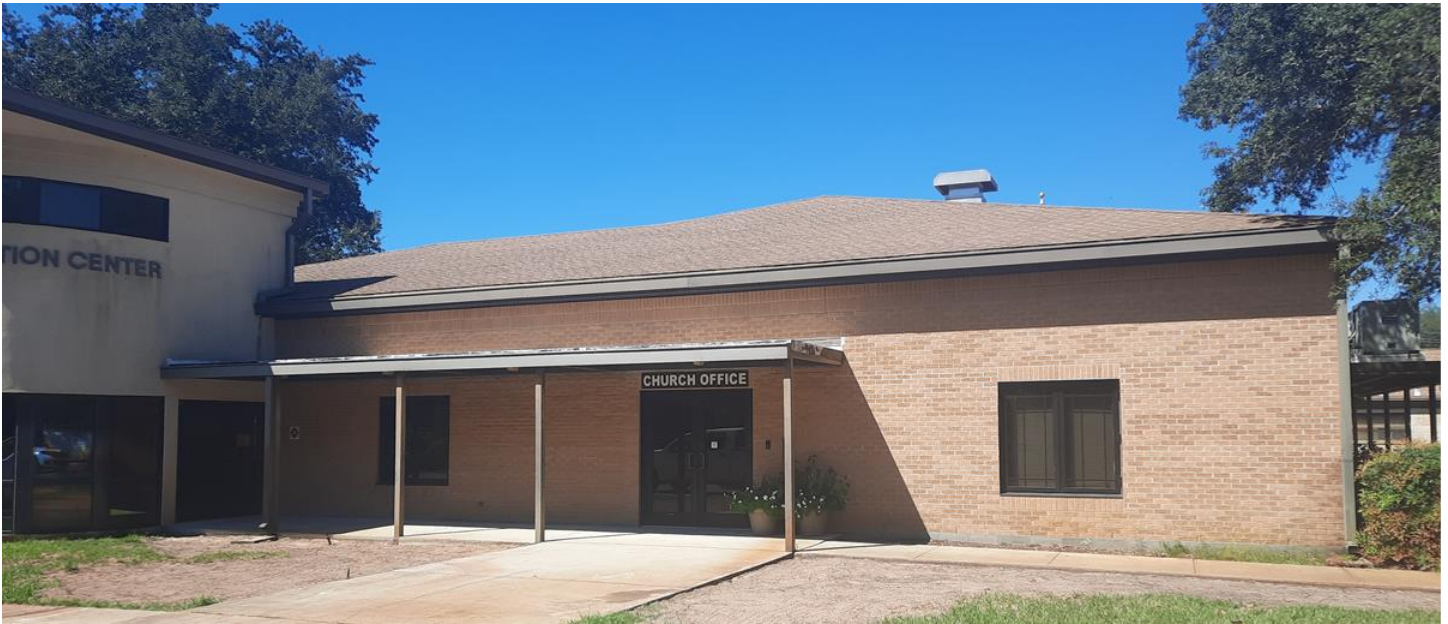
Bushes have been removed by the office awaiting sod.
