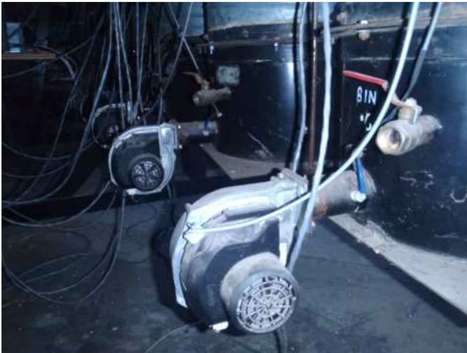
Figure 3-2. Centrifugal fan on each bin.
