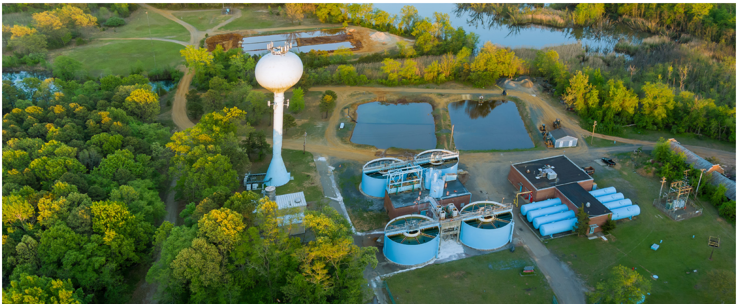
Aerial view of a wastewater treatment facility.
