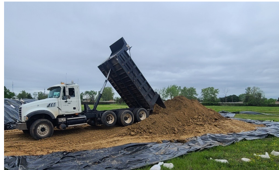
Truck unloading imported clean fill soil
