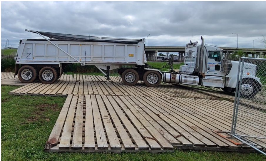
Large truck loaded with contaminated soil, with cover
