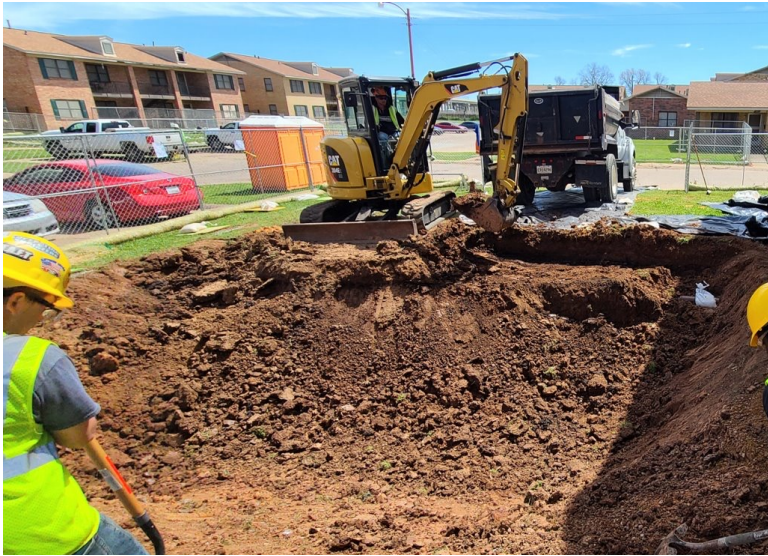
Small truck being loaded with excavated soil
