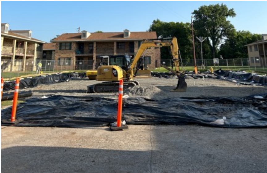
Placing clean backfill
