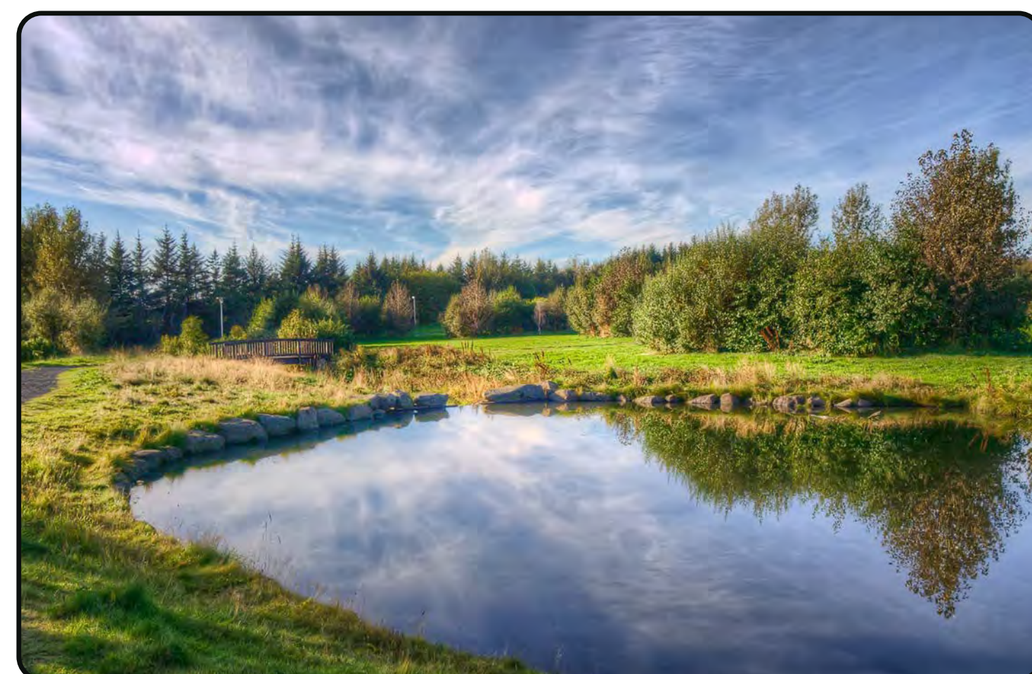
DETENTION POND Provide Stormwater Management While Offering Unique Water Experiences
