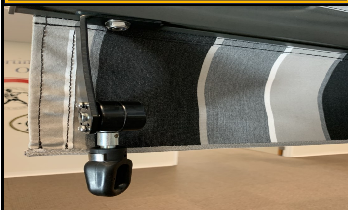
Install Drive End Bracket Leaving Bolt Loose
