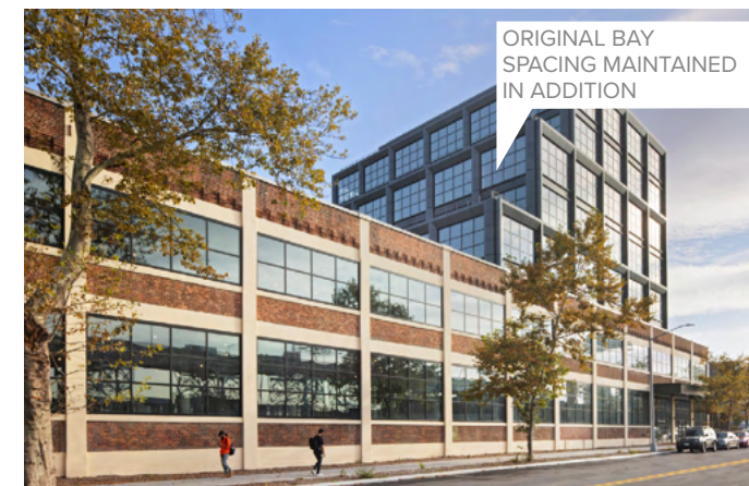
Adaptive Reuse + Vertical Addition Gantry Point Office Mid-Rise - Queens, NY Source: STUDIOS Architecture
