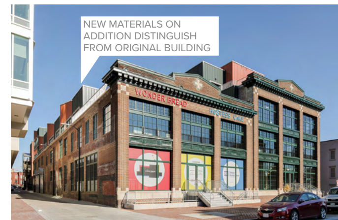
Façade Renovation + Lot Infill Wonder Bread Factory Commercial / Office Building - Washington, DC Source: Dewberry + Douglas Development
