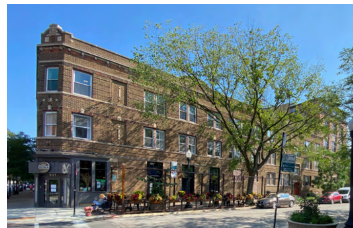
Mixed-Use Apartment Buildings (3-4 Story) 5101 N Clark Street - Ground floor restaurant and apartments above
