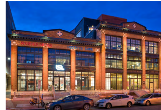
Source: Wonder Bread Factory, Washington, DC (Douglas Development + R2L Architects)
