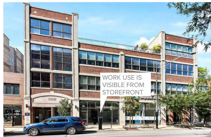
Live-Work Lofts Converted warehouse building into lofts
