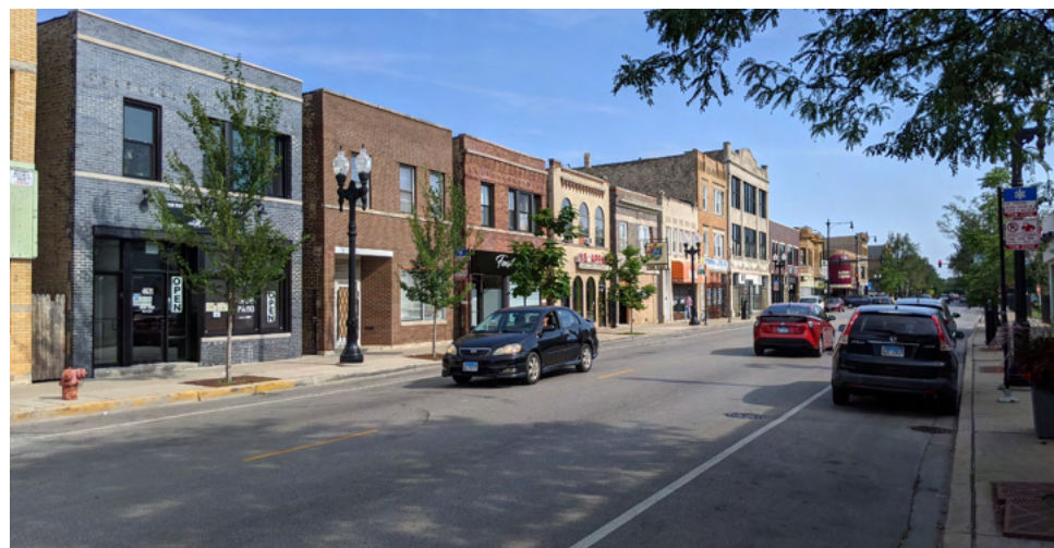
Historic Façade and Consistent Building Heights
