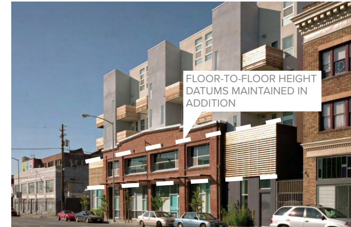
Façade Renovation + Lot Infill Folsom + Dore Affordable Housing - San Francisco, CA Source: David Baker + Partners
