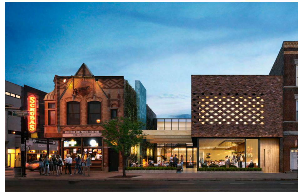
Source: Tied House, Schubas, Chicago, IL (Gensler)
