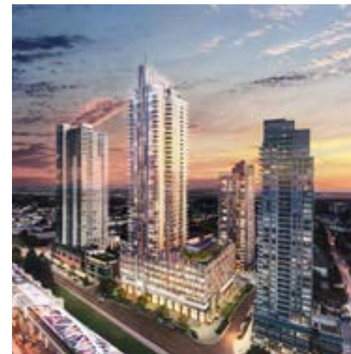
METROTOWN Sun Towers and future projects
