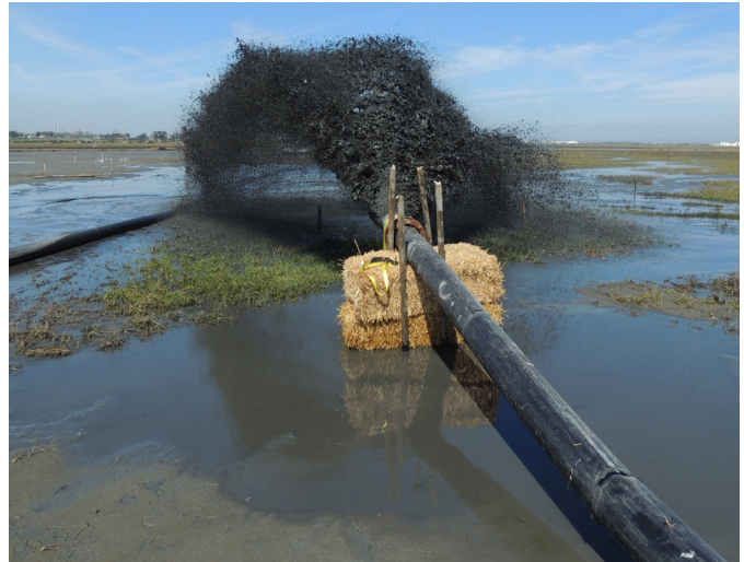
▲ Figure 5: 'Rainbow' spray of sediment onto the augmentation site. Photo credit: Rick Nye.
