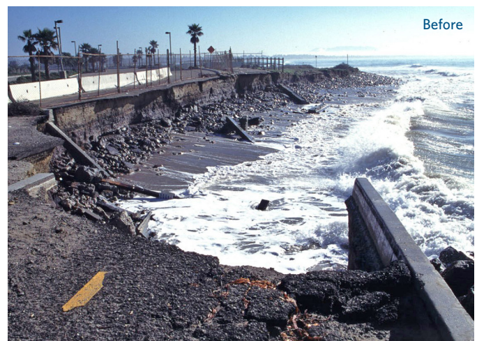
▲ Figure 9: Project site before landward realignment of built infrastructure and restoration of the dunes and beach. The bike path and parking lot were built on fill in 1989 and eroded within 2 years. Photo credit: Paul Jenkin.
