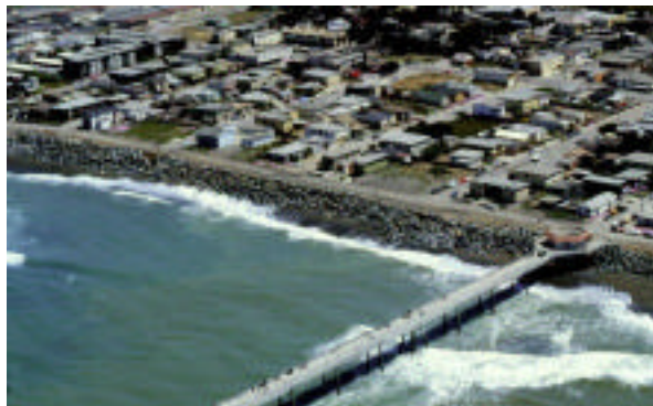
Figure 11. The placement of riprap to protect this low bluff south of San Francisco has led to the loss of beach due to a combination of placement loss and passive erosion.
