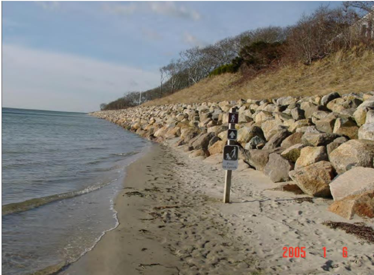
Figure 5-1: Loss of Beach Access Due to Revetments
