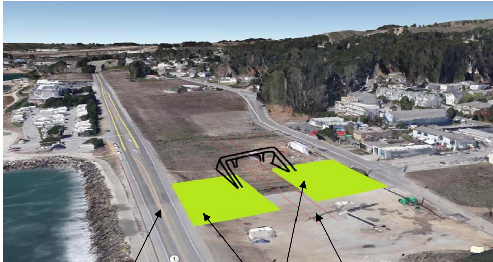
Existing roadway to be converted to parking
