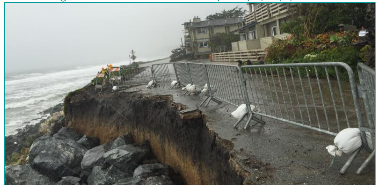
Eroded segment of Mirada Rd with temporary riprap protection.
