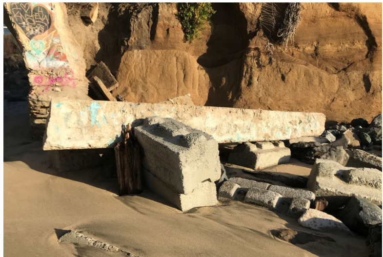
Figure 2. Southerly abutment of the existing concrete arch bridge.
