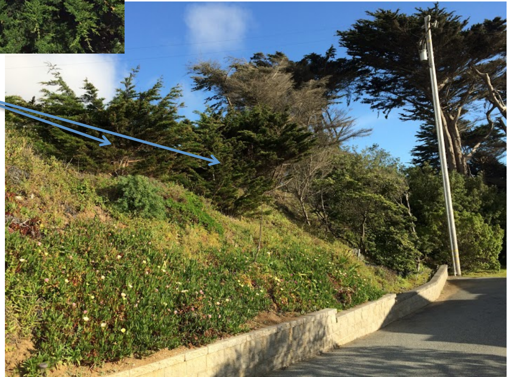
View from entry road to 200 – 14 th St below Hwy 1 embankment
