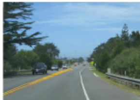
Painting existing median helps to provide traffic calming
