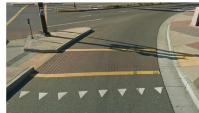
Figure 5: Advance Yield Markings at a Pedestrian Crossing
