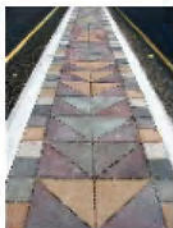
RAISED MEDIAN WITH DECORATIVE PAVERS
