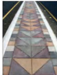
RAISED MEDIAN WITH DECORATIVE PAVERS Proposed raised median provides traffic calming and refuge for crossing pedestrians
