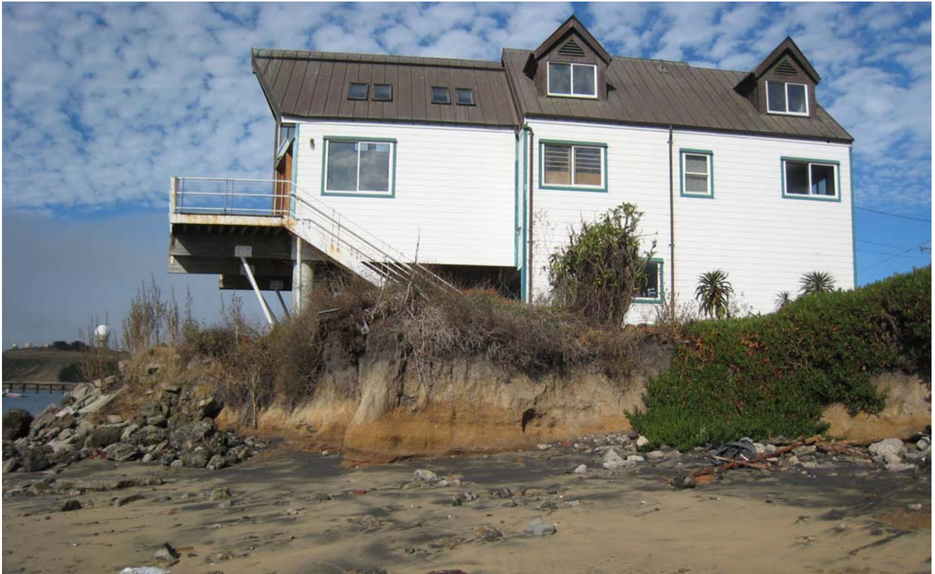
Extensive erosion of parcels next to riprap
