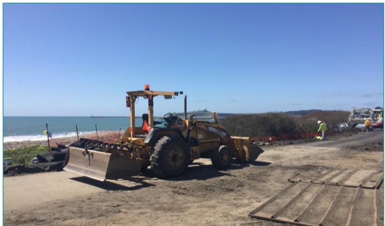
Construction and repair at Surfer's Beach.
