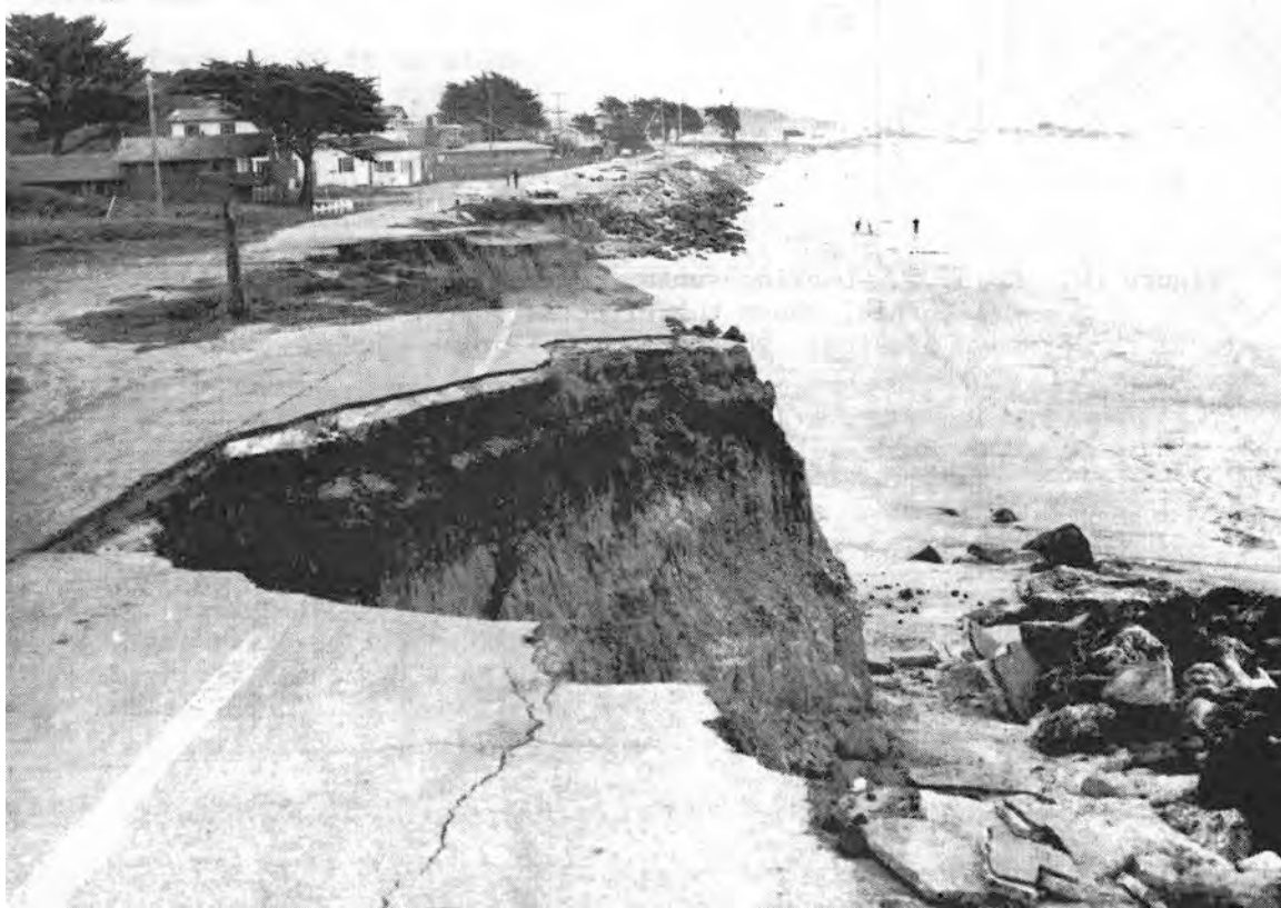
Figure 10: 1971 photograph of Mirada Road looking south from near the root of the East Breakwater. Riprap can be seen along the sea cliff starting at about the white house and going south. Photograph by K. Lajoie, USGS.
