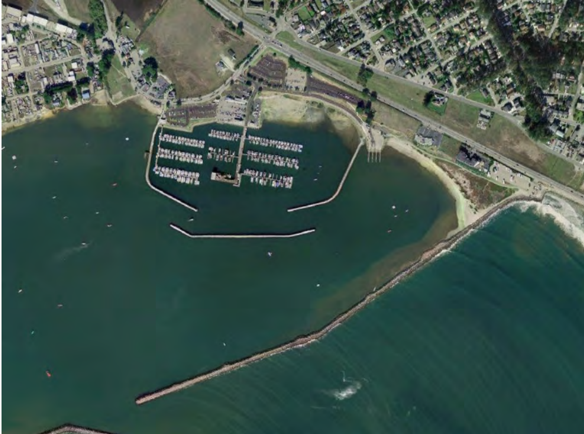
Figure 7: East end of Pillar Point Harbor showing the East Breakwater, inner breakwaters, and inner sand wedge adjacent to the root of the East Breakwater.
