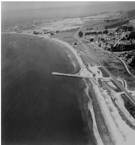
Figure 8: Sediment wedge inside the East Breakwater December 1959 (SPN archives).
