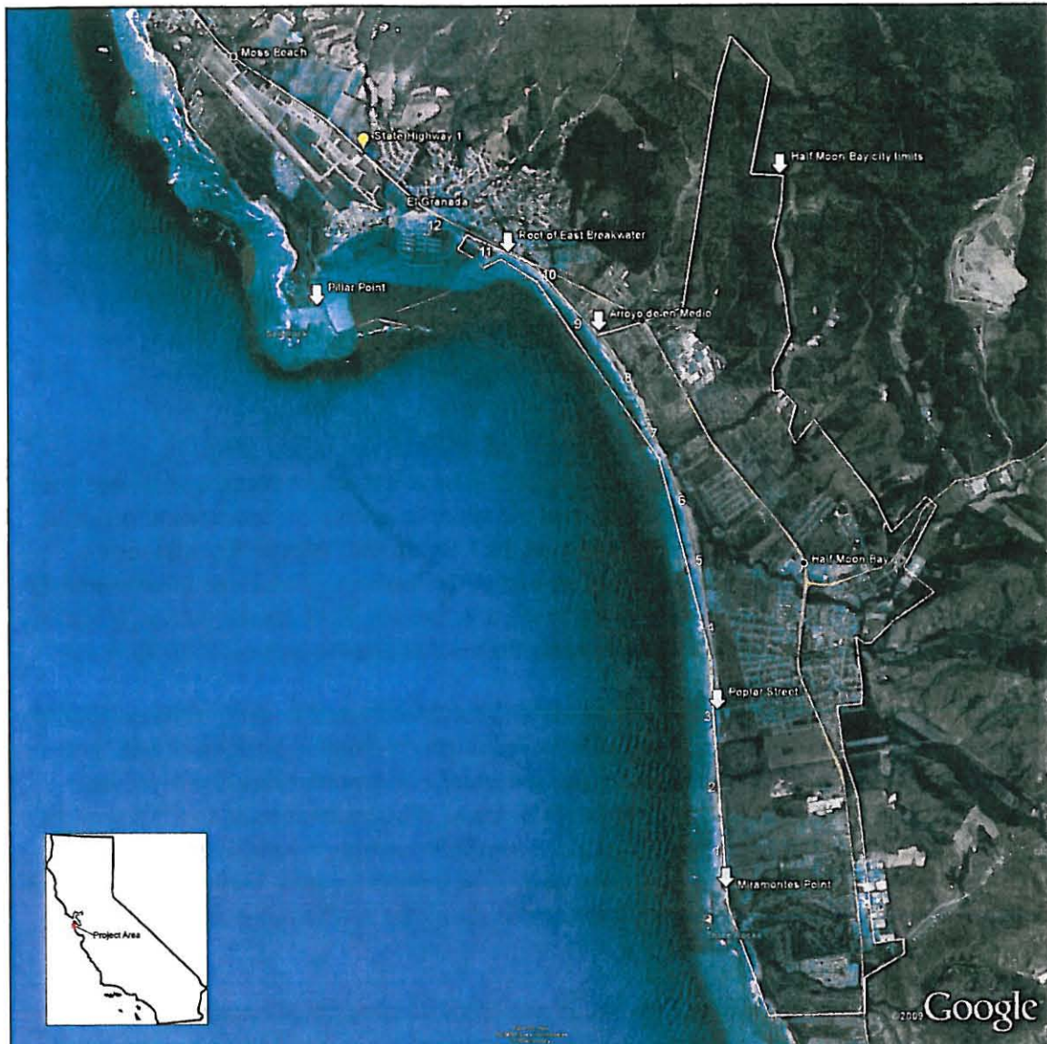
Figure 1: Google Earth image of Half Moon Bay. Arrows mark the bounding headlands (Pillar Point and Miramontes), the southern end of the urbanized area (Poplar Street), and the extent of the project area (Root of the Breakwater to Arroyo de en Medio). Station numbers for Table 1 are shown in white.
