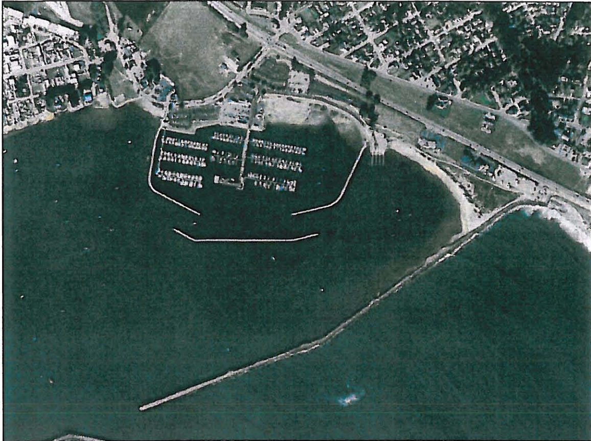
Figure 5: East end of Pillar Point Harbor showing East Breakwater, inner breakwaters, and inner beach adjacent to the root of the East Breakwater.
