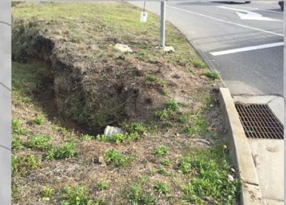
STORM DRAIN INLET AT SOUTHEAST CORNER OF CORONADO STREET AND HIGHWAY 1
