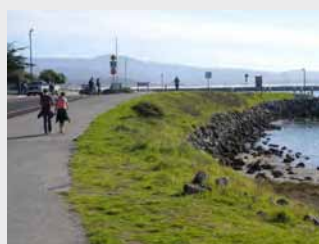
Pillar Point Harbor path
