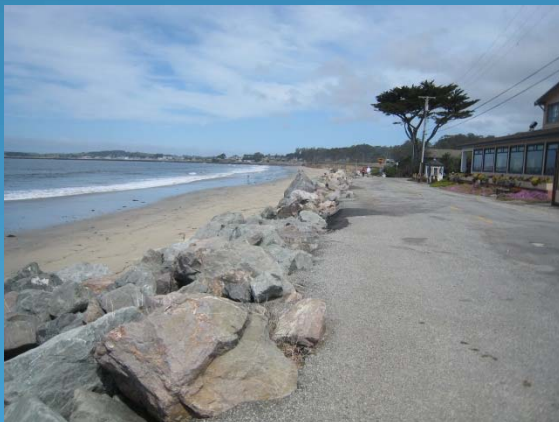
Miramar - Mirada Road Riprap
